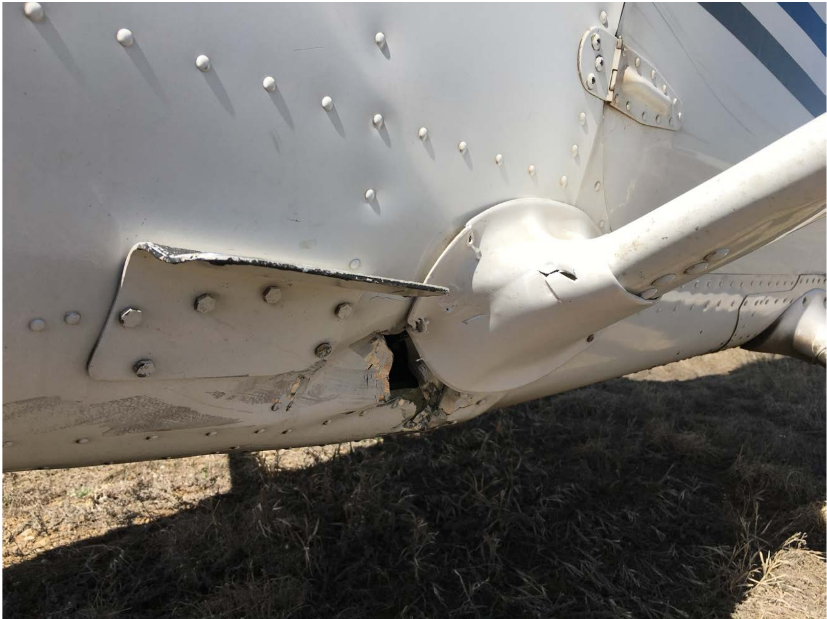
Photo 1 – View of damage to the lower left side longeron (Courtesy of FAA)
