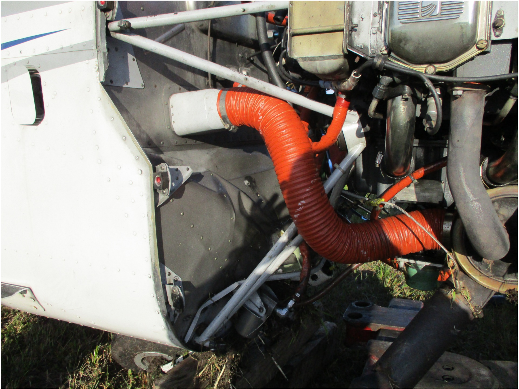
Photo 2 – View of buckled firewall
