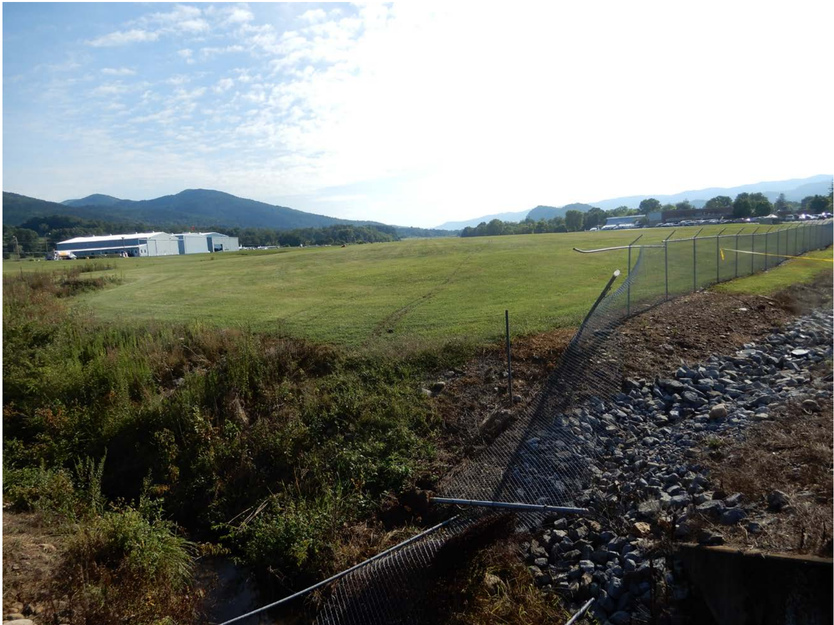
Photo 17 – Creek Bed and Airport Perimeter Fence (NTSB Photo)
