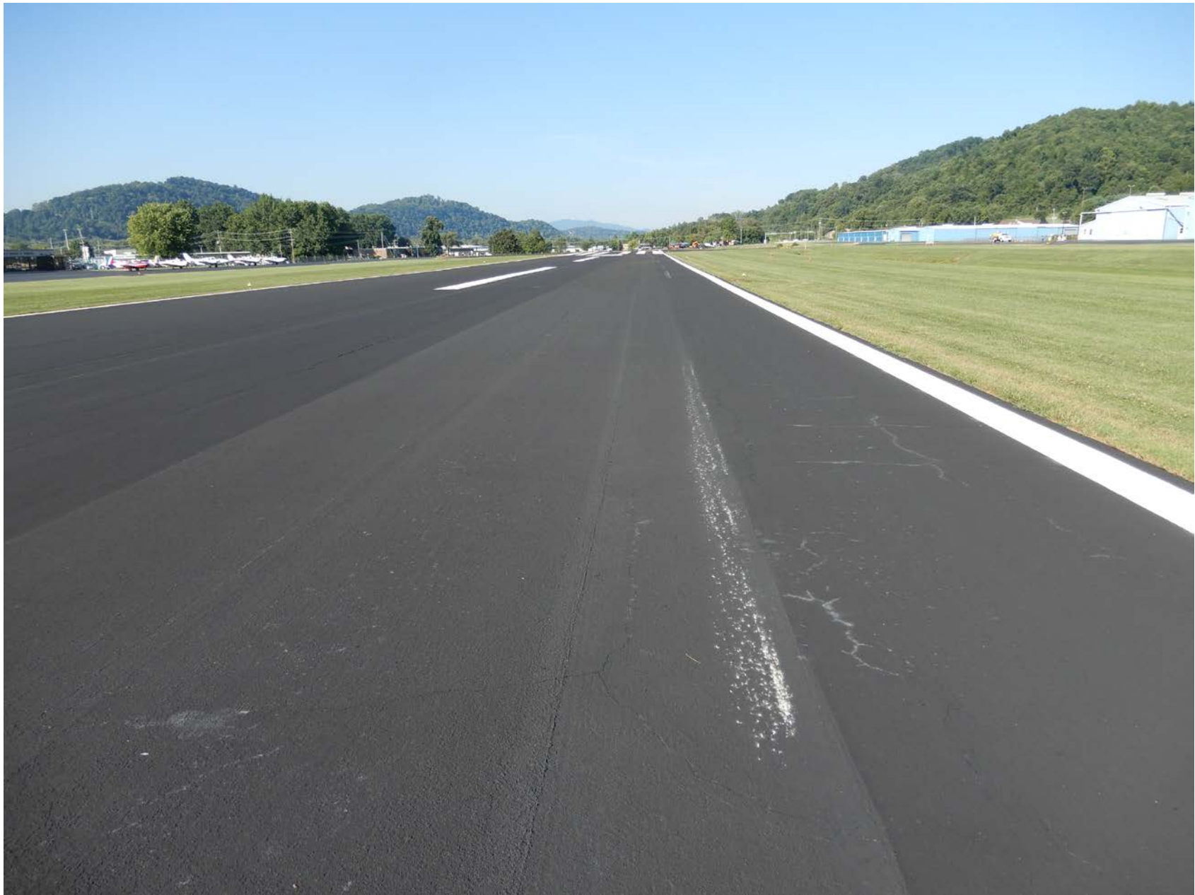
Photo 15 – Point of Initial Right Wing Tip Impact on Runway (NTSB Photo)
