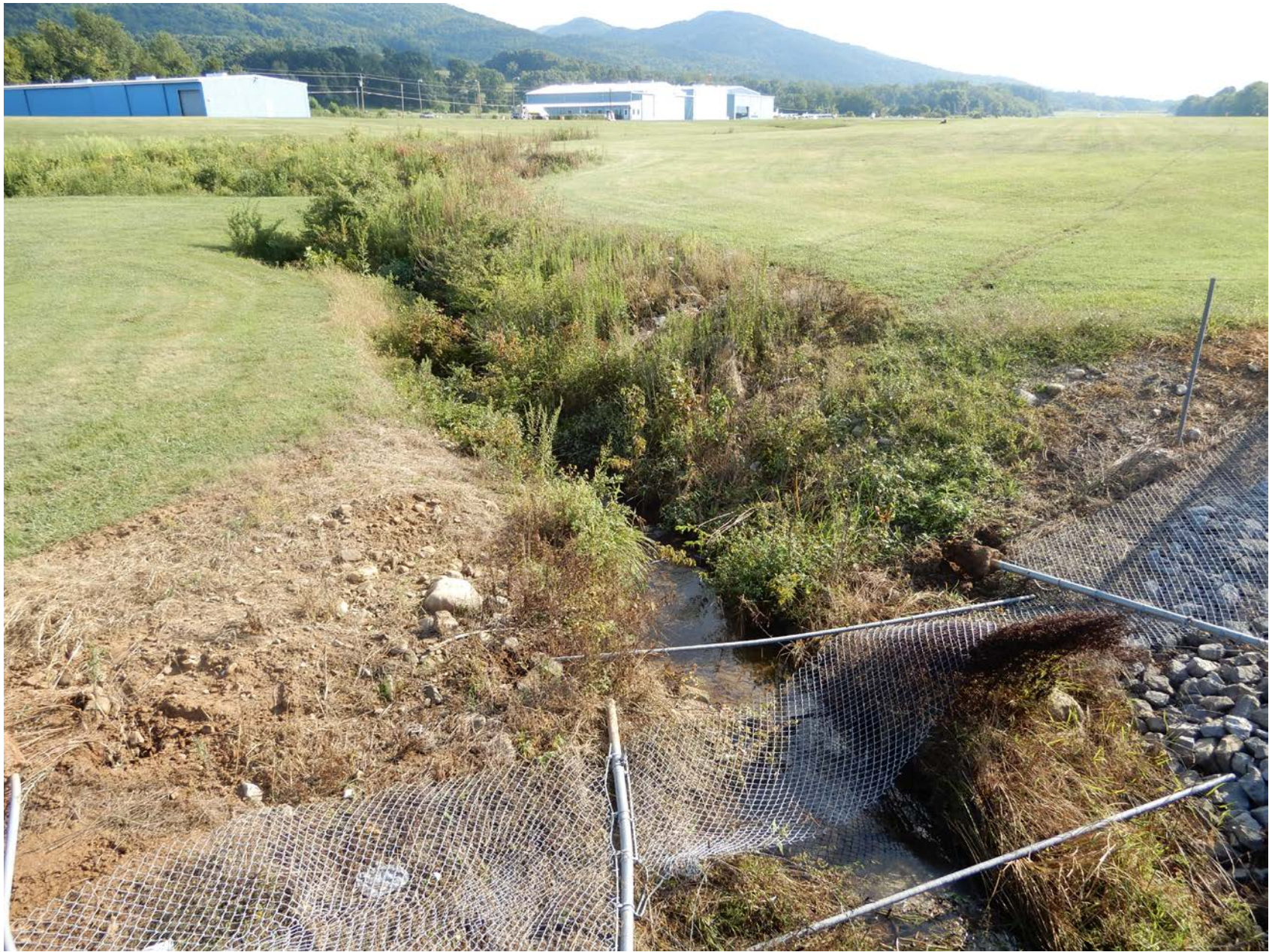
Photo 18 - Creek Bed and Airport Perimeter Fence (NTSB Photo)
