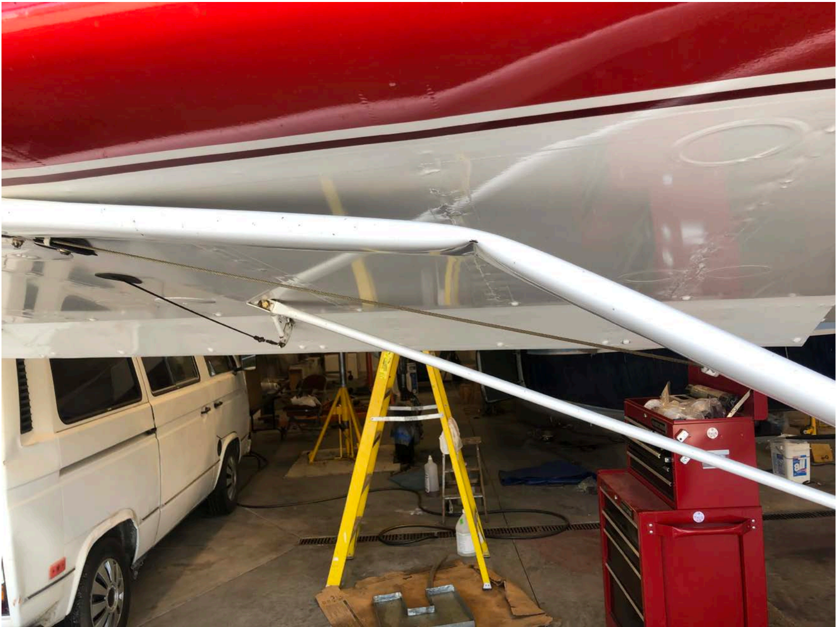
Photo 2 - Photo of the damaged right lift strut. Photo courtesy of McLarens Insurance Company.
