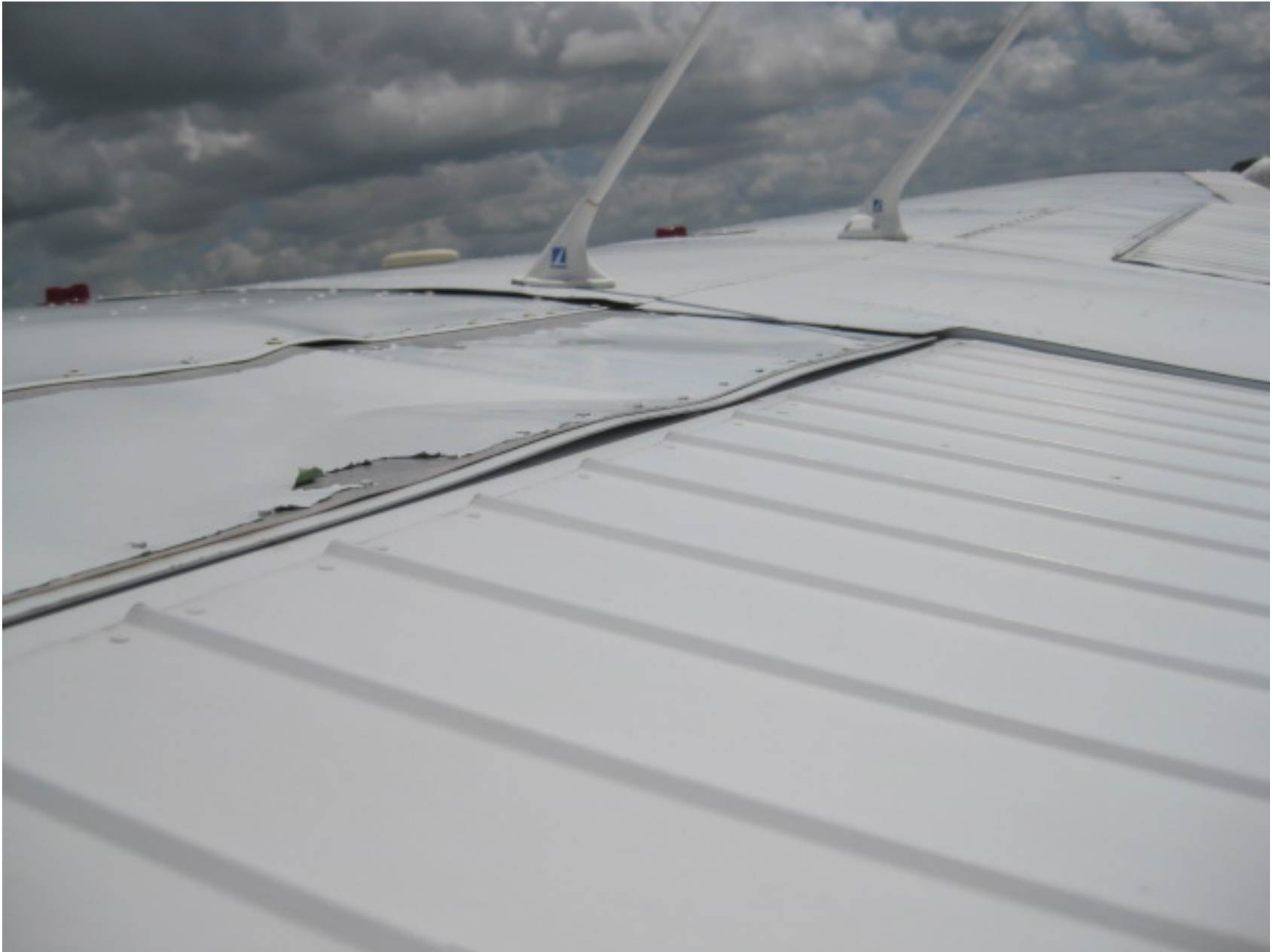
Photo 3 – Left Wing Damage (Photo Courtesy of FAA)
