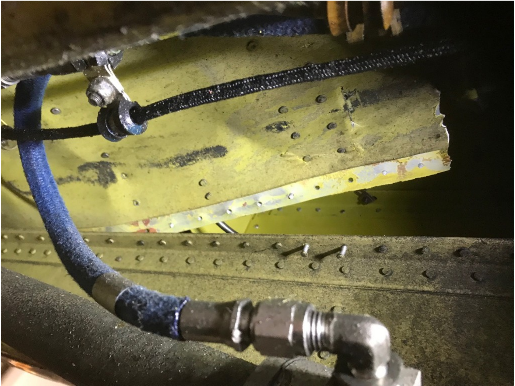
Photo 3 – Area Above Nose Landing Gear (Photo Courtesy of FAA)
