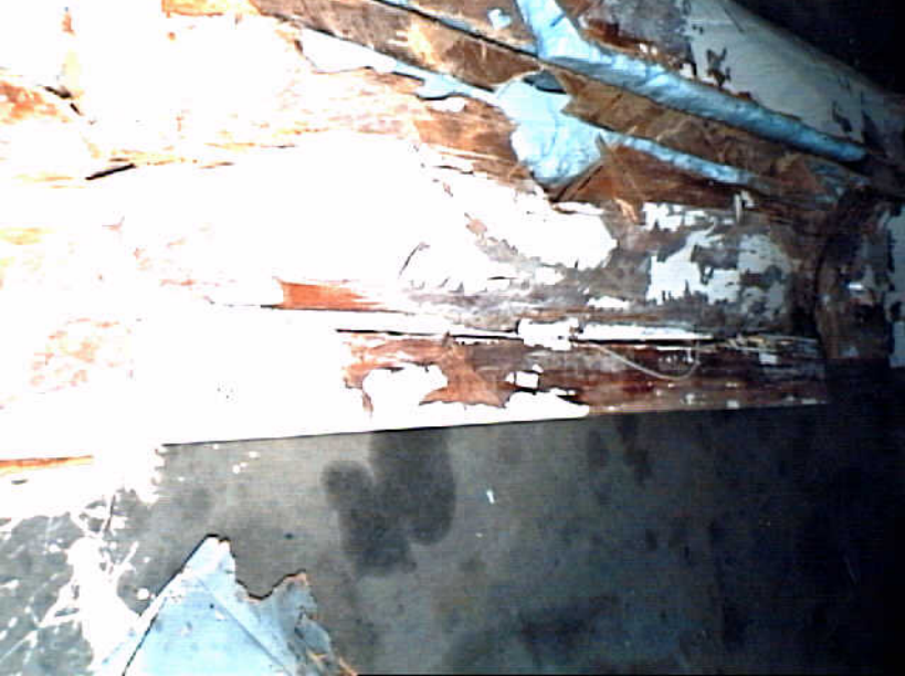
Photo 7. Right wing structure.
