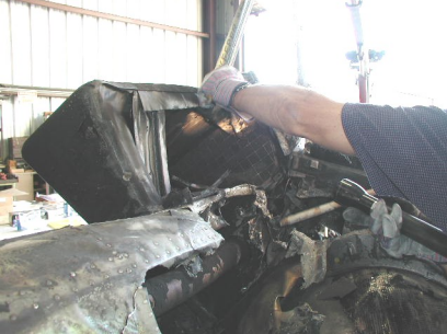
Photo 7. Plenum chamber (doghouse).
