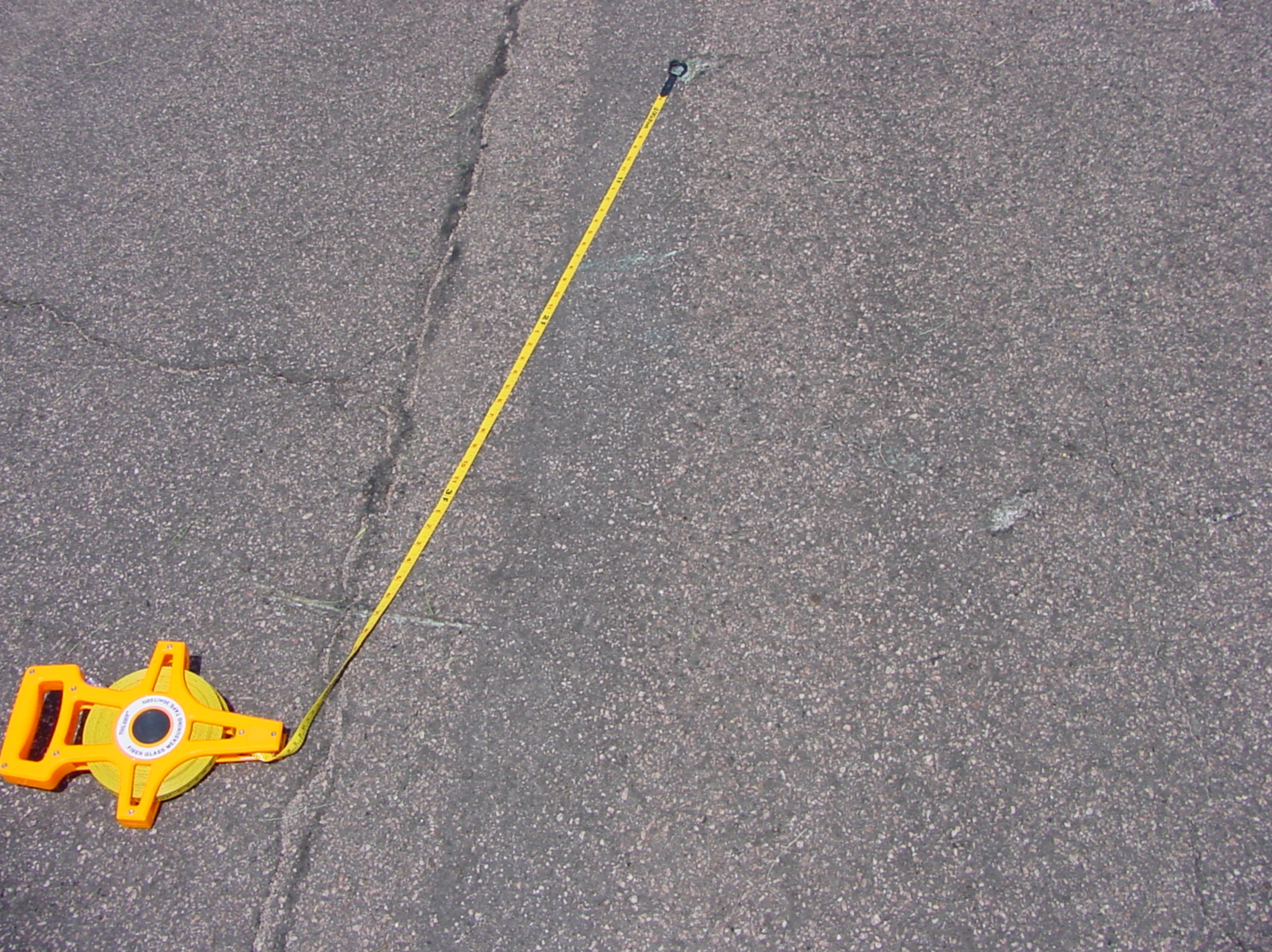
Photo 4. Marks in Taxiway Between Initial Impact Point and Main Wreckage
