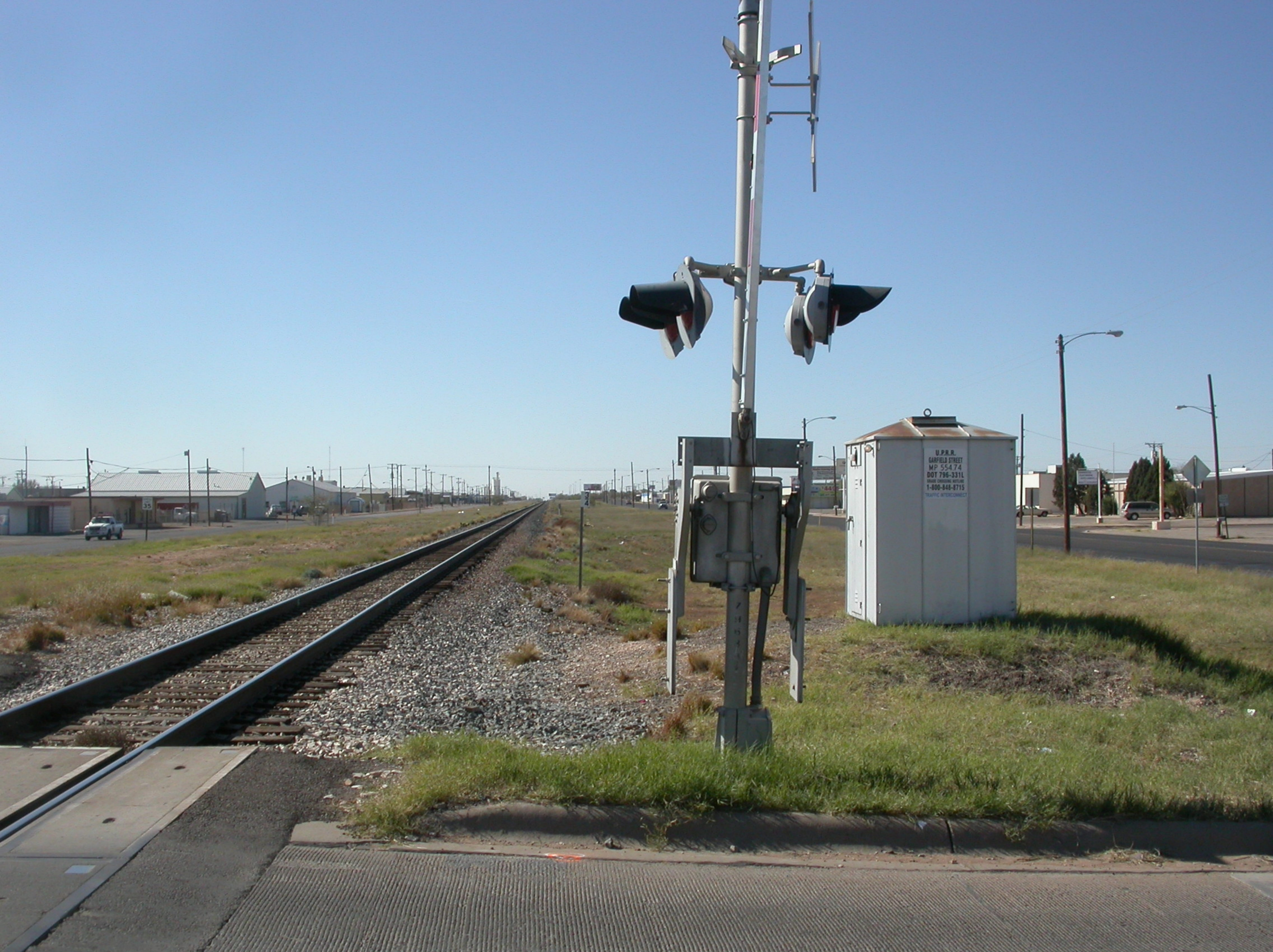
Photo 4: Westbound view of railroad tracks at the grade crossing.
