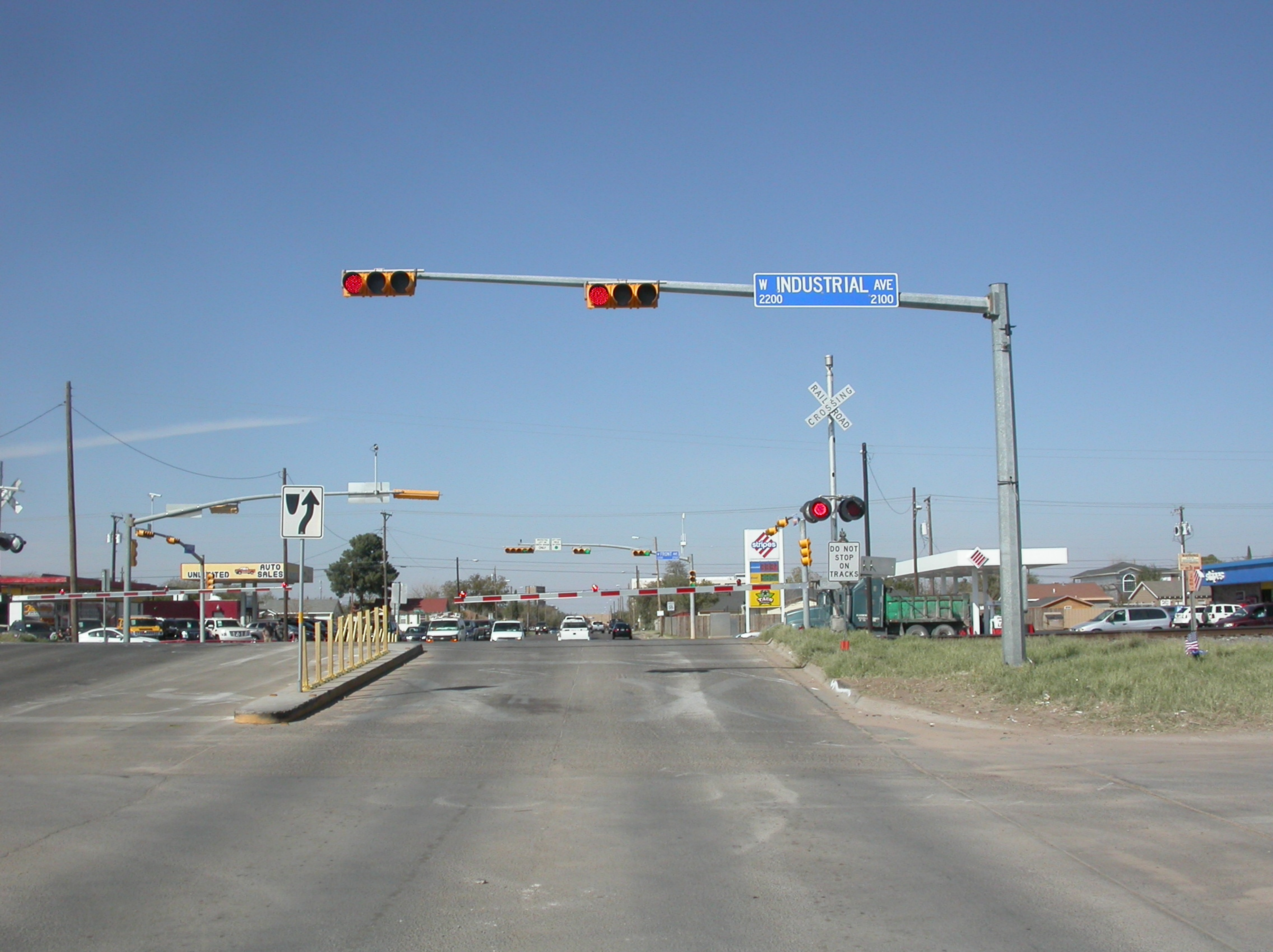
to 3: Northbound view of the S. Garfield Street approaching the grade crossing, showing the traffic signals and grade crossing signals and gates.
