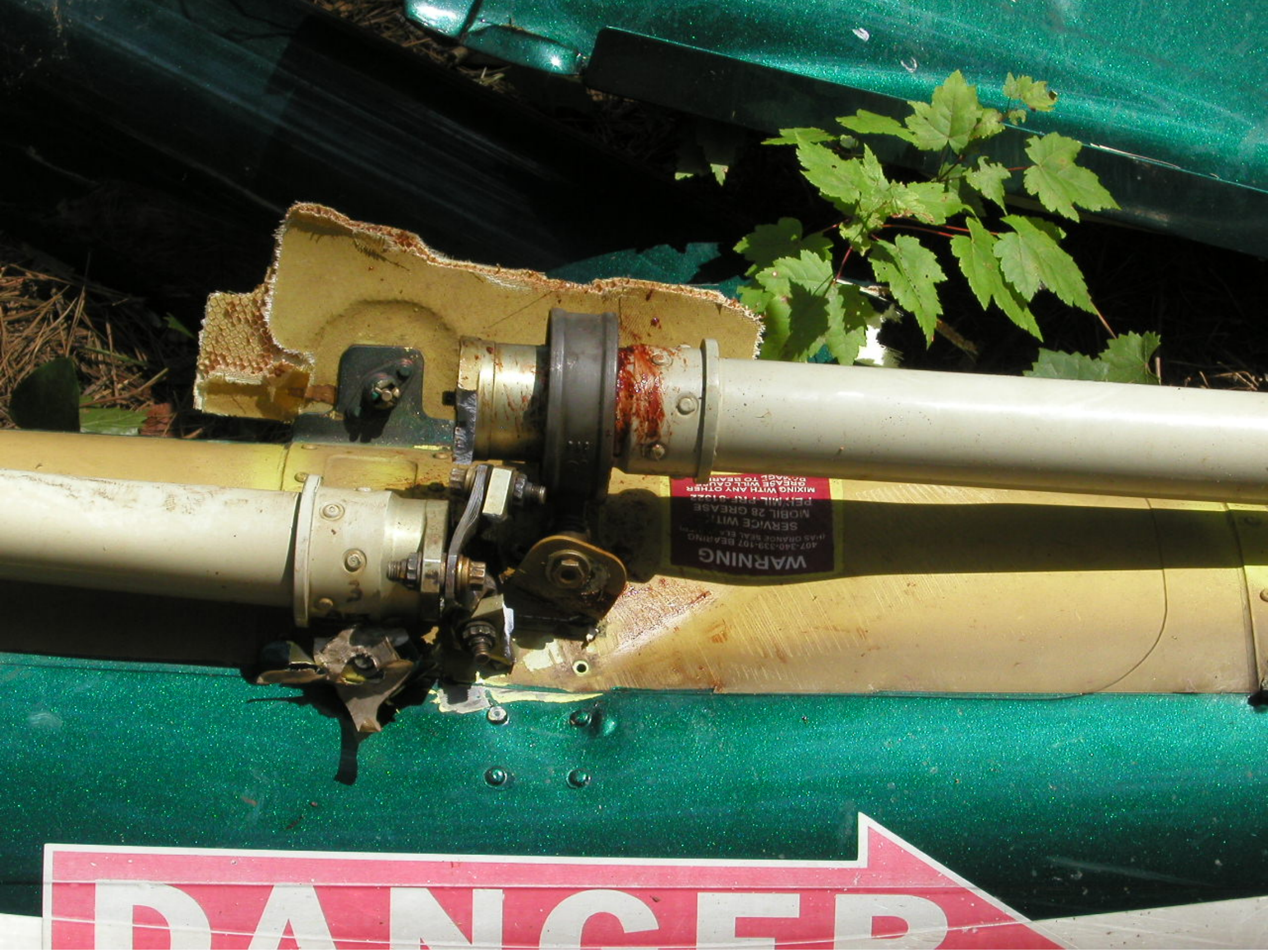
Photo 23. #6 Tail Boom Hangar Bearing
