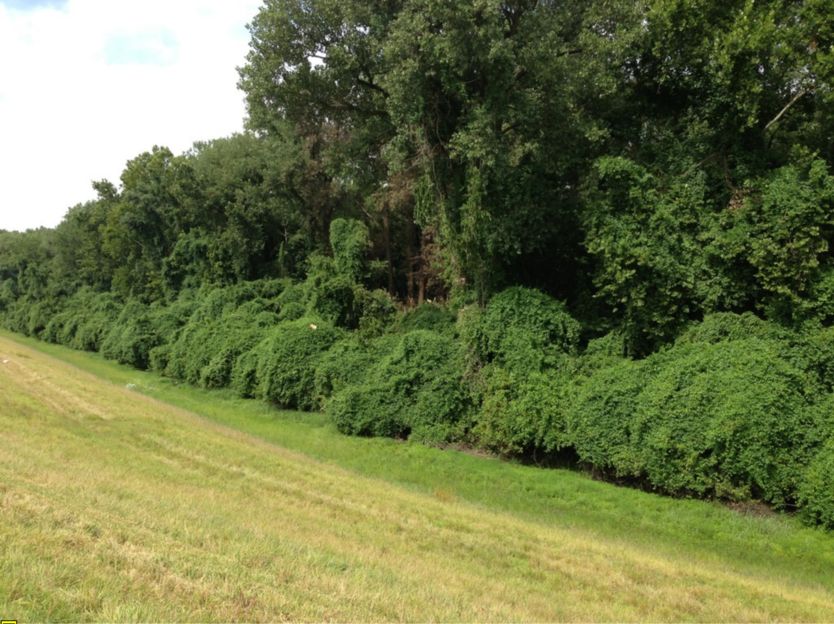
Photo 2. View of the woods from the top of the dike.
