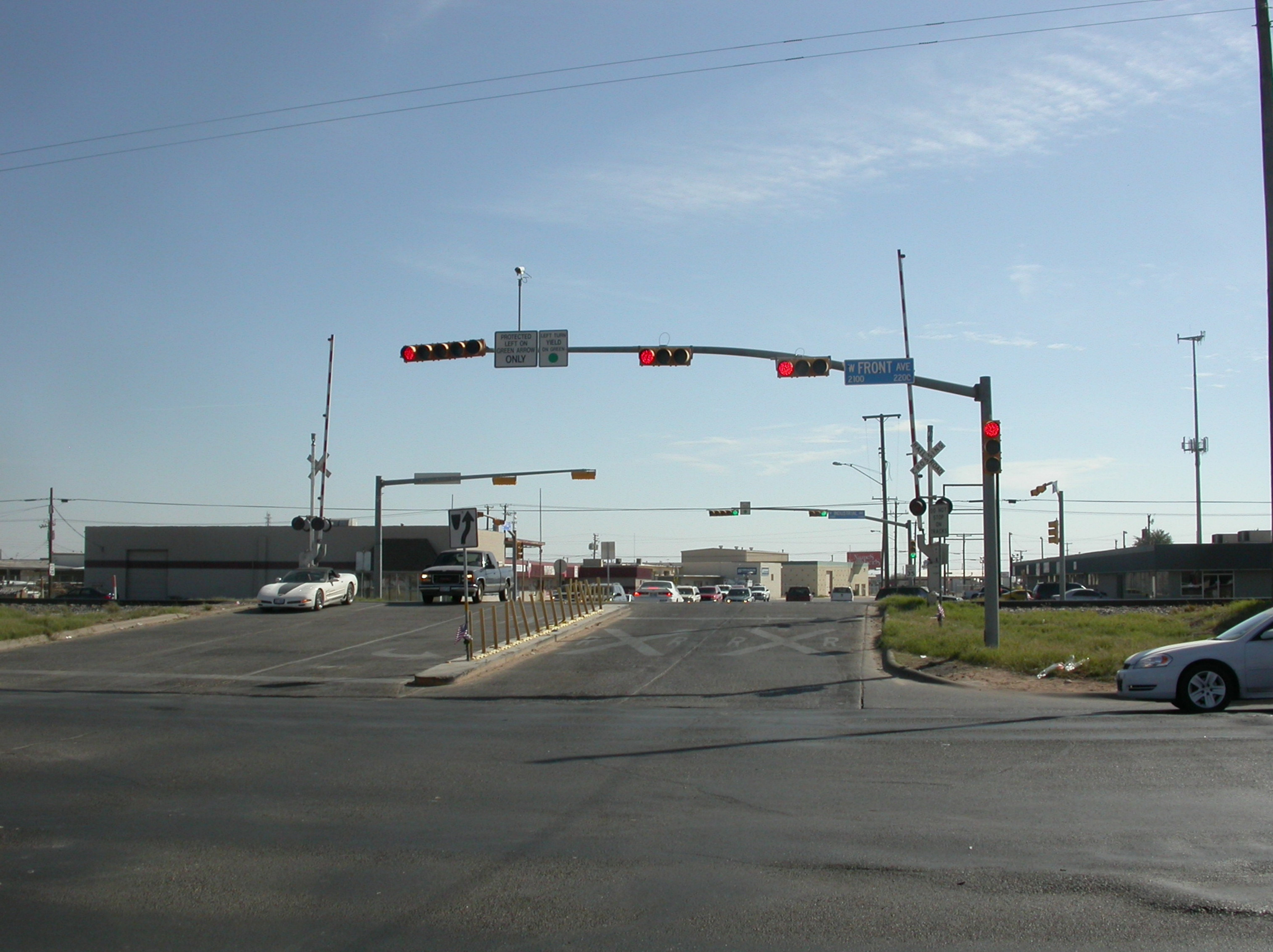
Photo 2: Southbound view of S. Garfield Street approaching the grade crossing.
