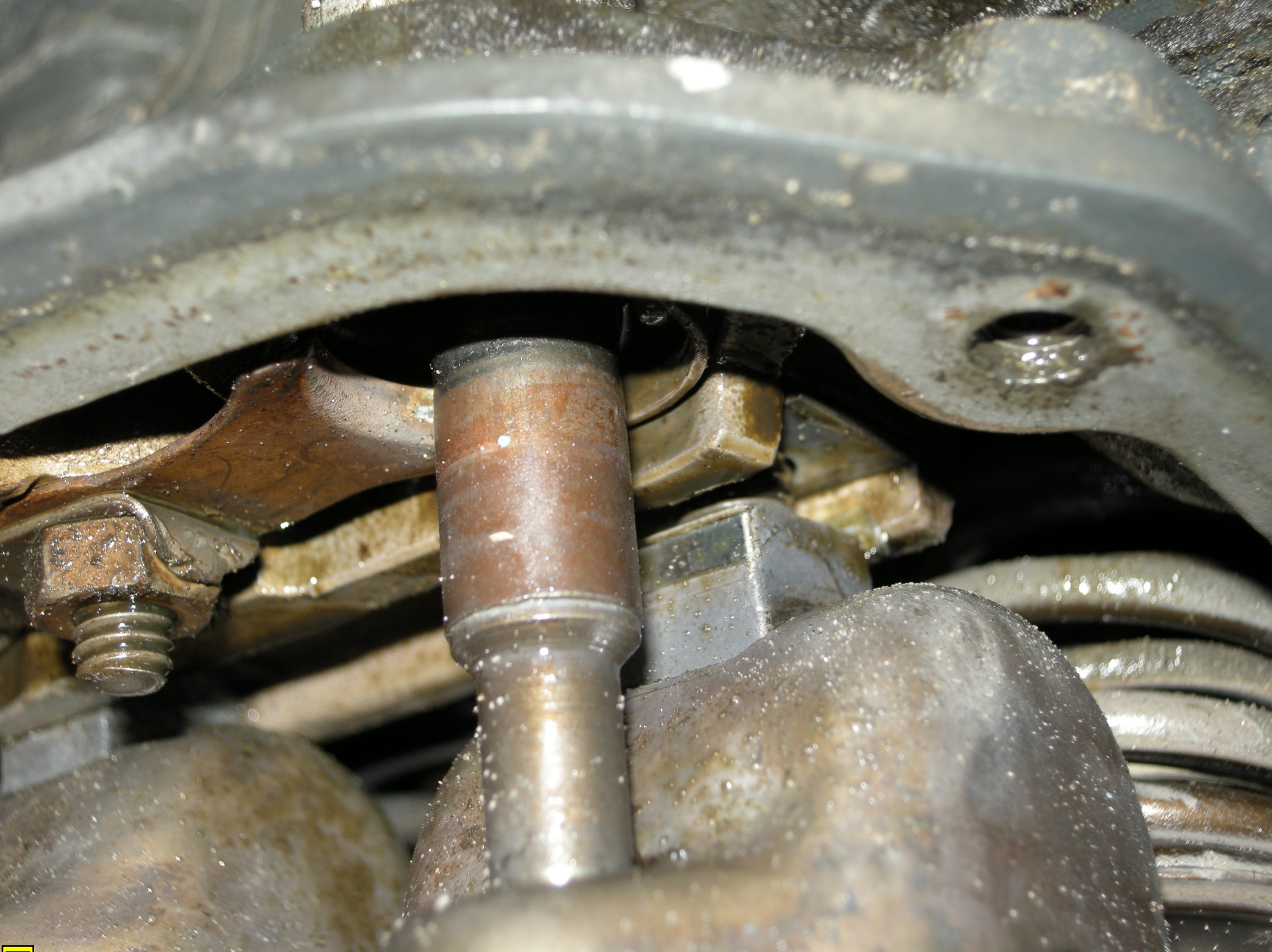
Photo 2: Gap in the Rocker Arm Fulcrum, Showing the Stud.
