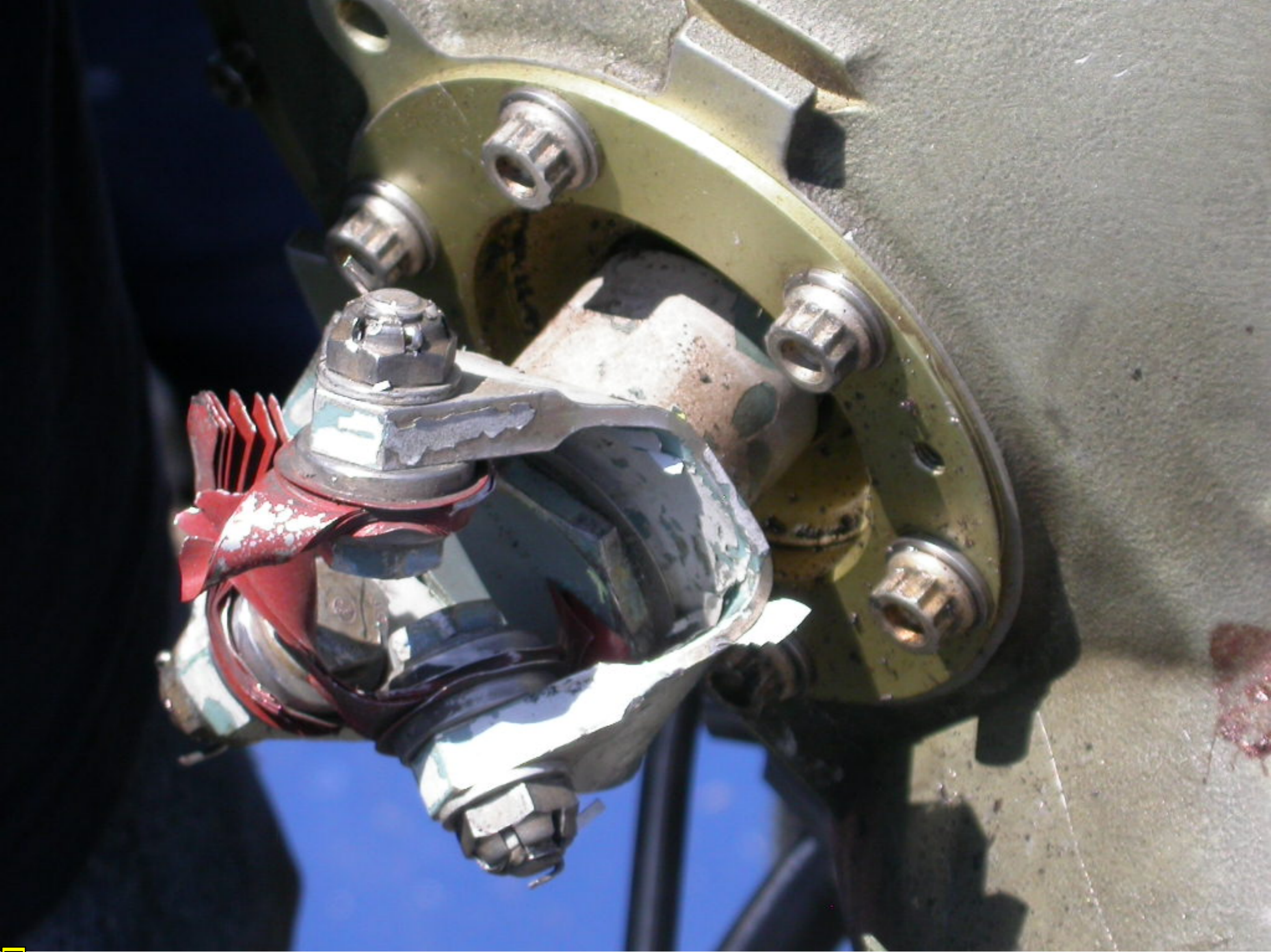
Photo 12: Tail rotor drive shaft coupling on main transmission
