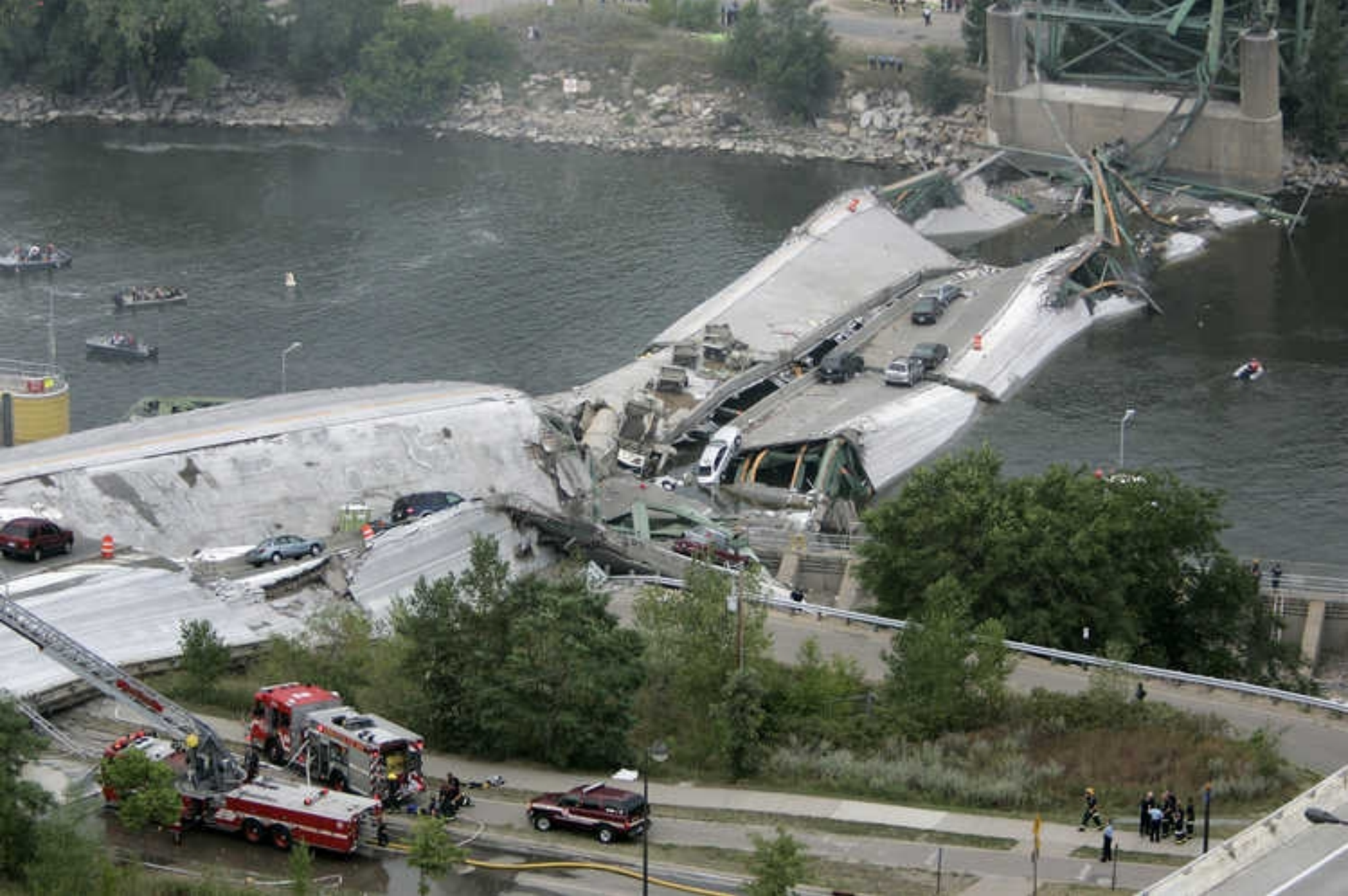
Photo 1. Overhead view of bridge in water looking north
