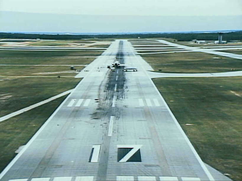
Photo 1. N927DA on runway 17 after coming to a stop. The oil streak is visible left of the runway centerline.
