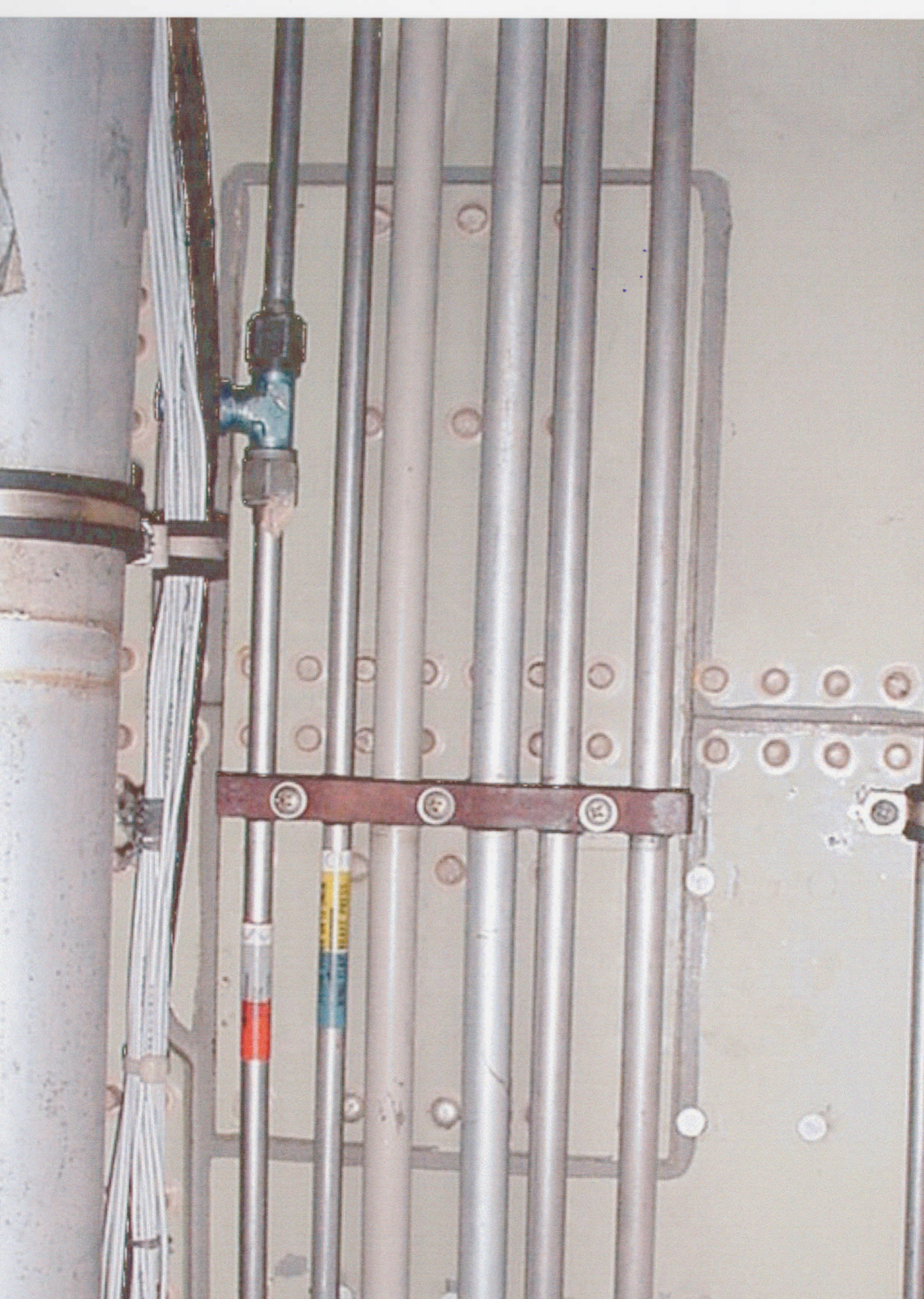
Photo 1. Center wing lower doubler installation.
