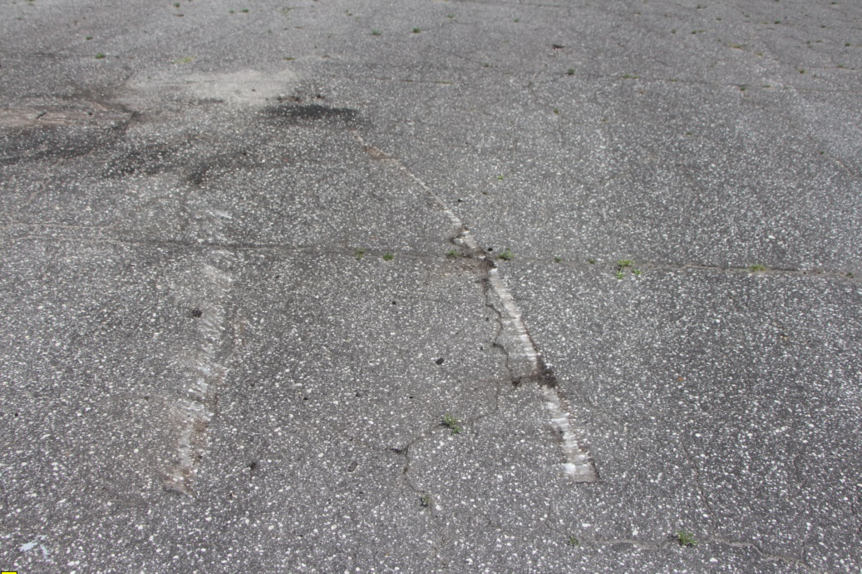
Photo 5: Ground Strikes from Rotor Blades.
