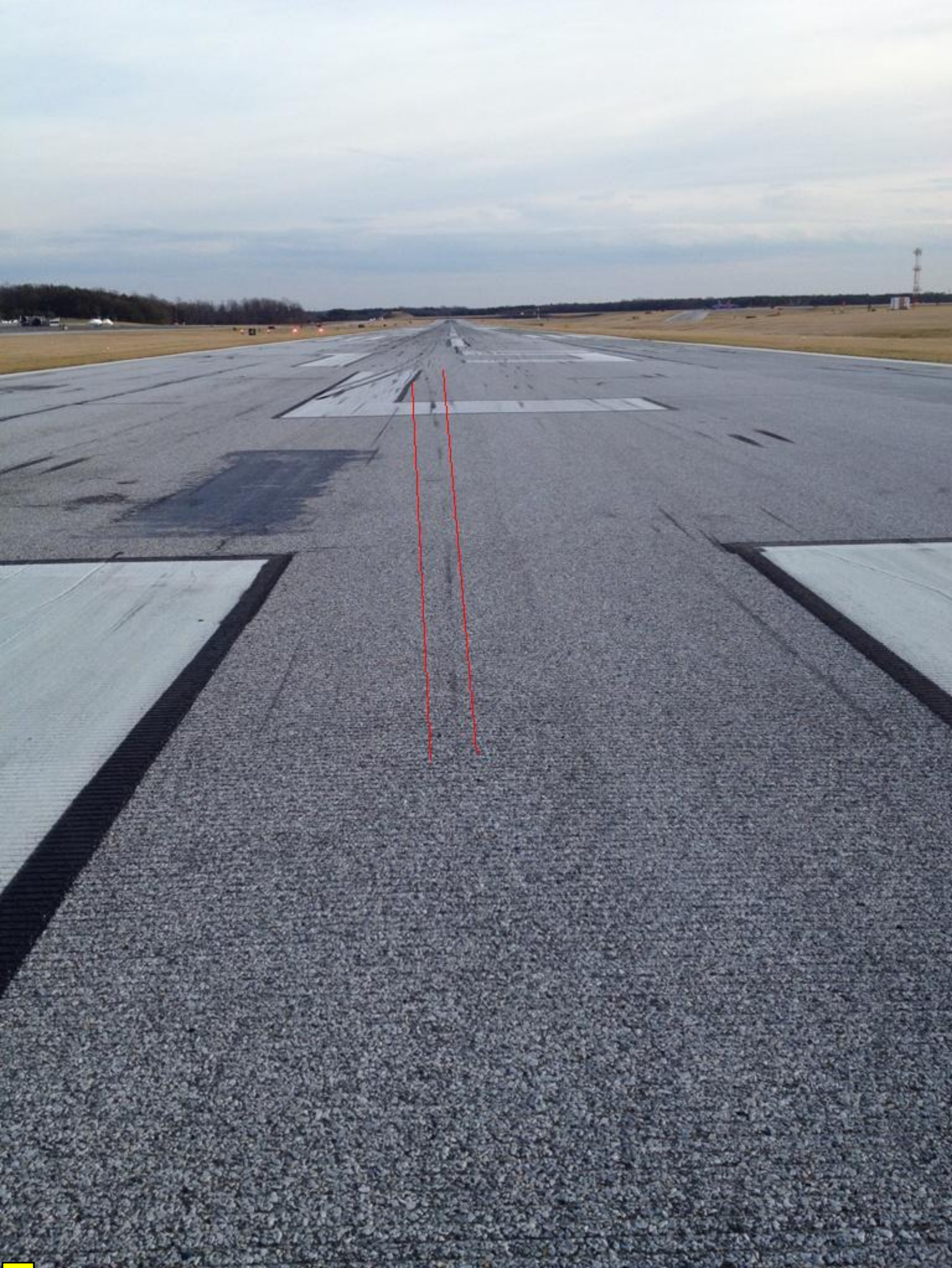
Photo: Right MLG Skid Marks (Photo Courtesy of FAA)
