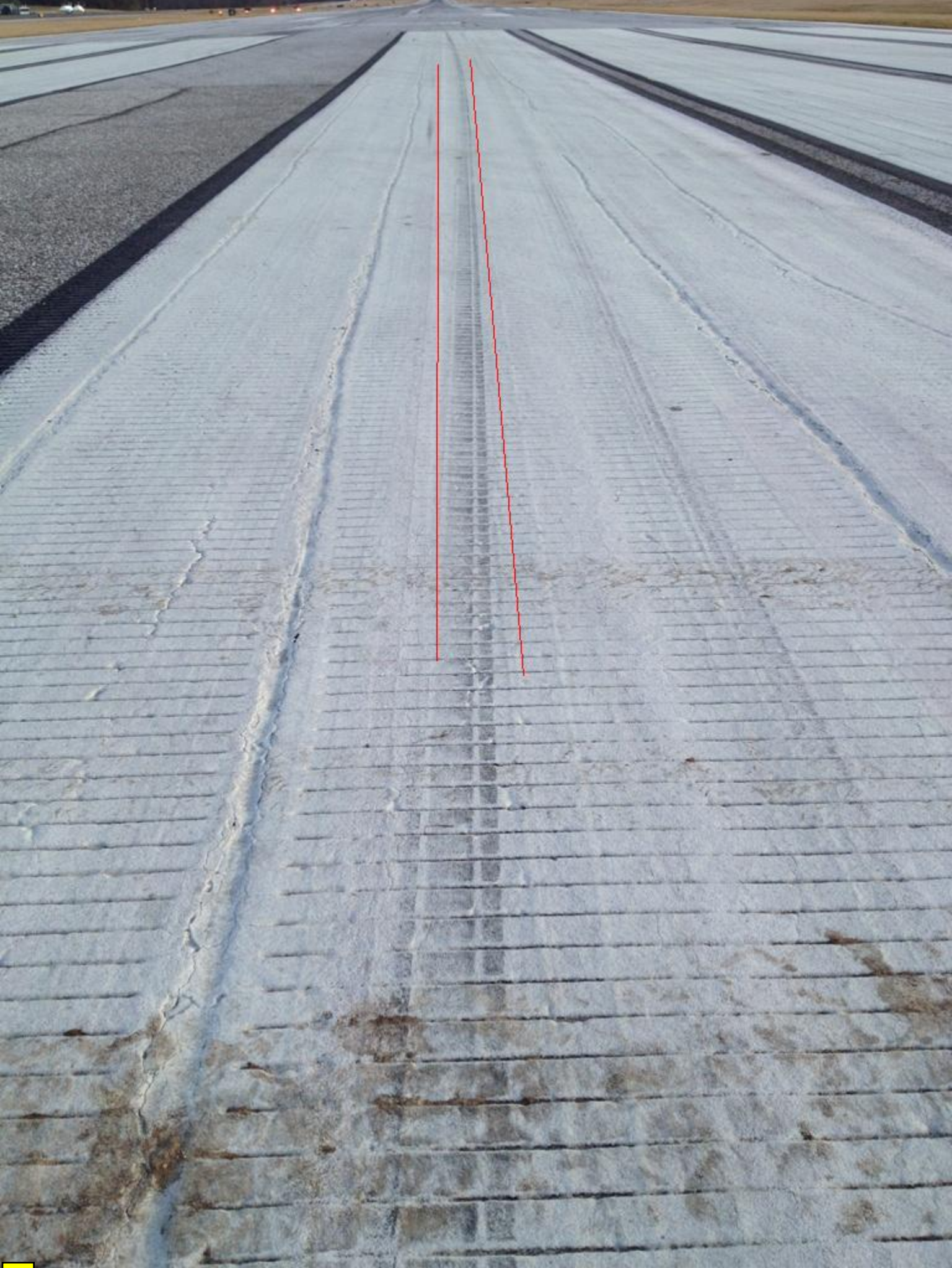
Photo: Left MLG Skid Marks (Photo Courtesy of FAA)
