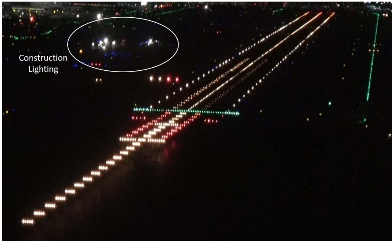
Figure 5: Construction Zone on runway 28L
