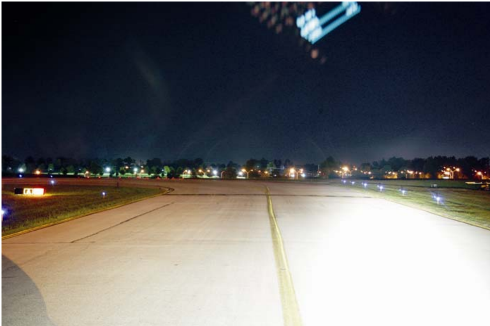
Photo 5: Taxiway "A" Approaching Runway 26
