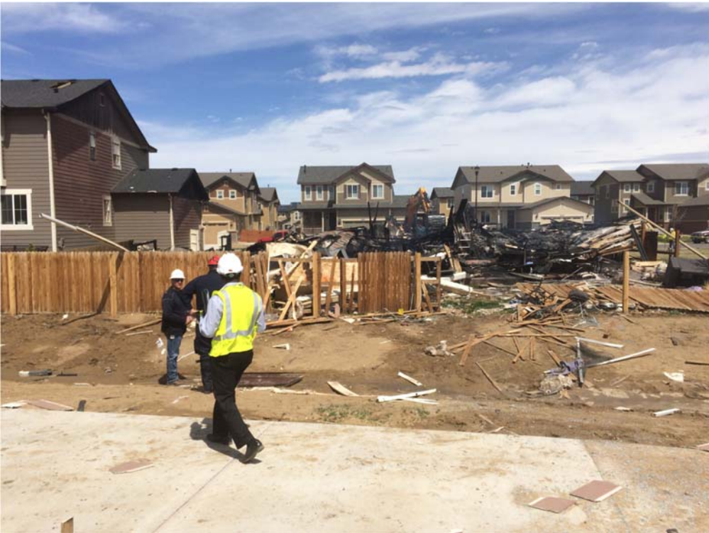
Figure 3: Explosion site from south side of property facing North.
