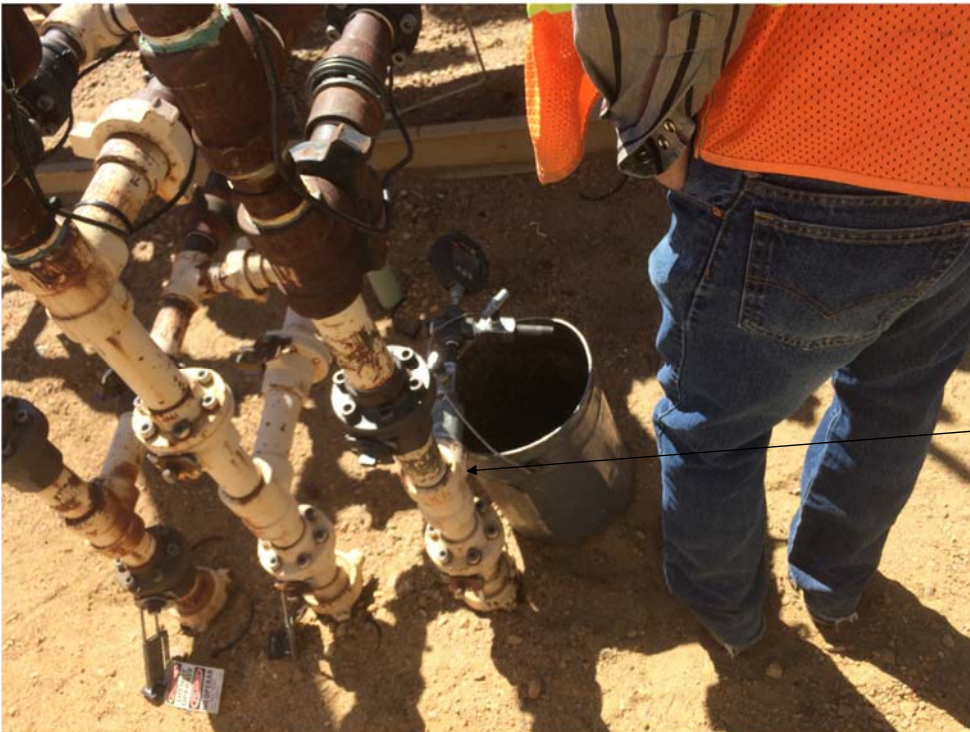
Figure 7: End of 2" flow line a separator facility with pressure gauge installed for hydrotest
