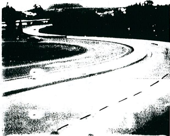
G/L 109 @ I-280 | 09-02-92 LOOKING DOWN STATION FROM INTX. OF SNEATH
