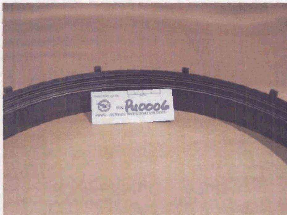
Photo no. 46 Another section view of the PT shroud shows the light rubs to the seal knives referred in photo no. 43 above.
