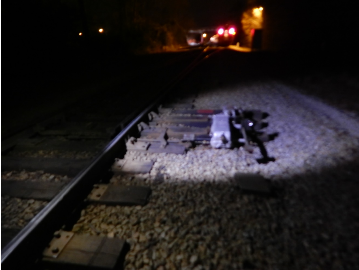
Figure 5. View of T21 switch at night with added light.
