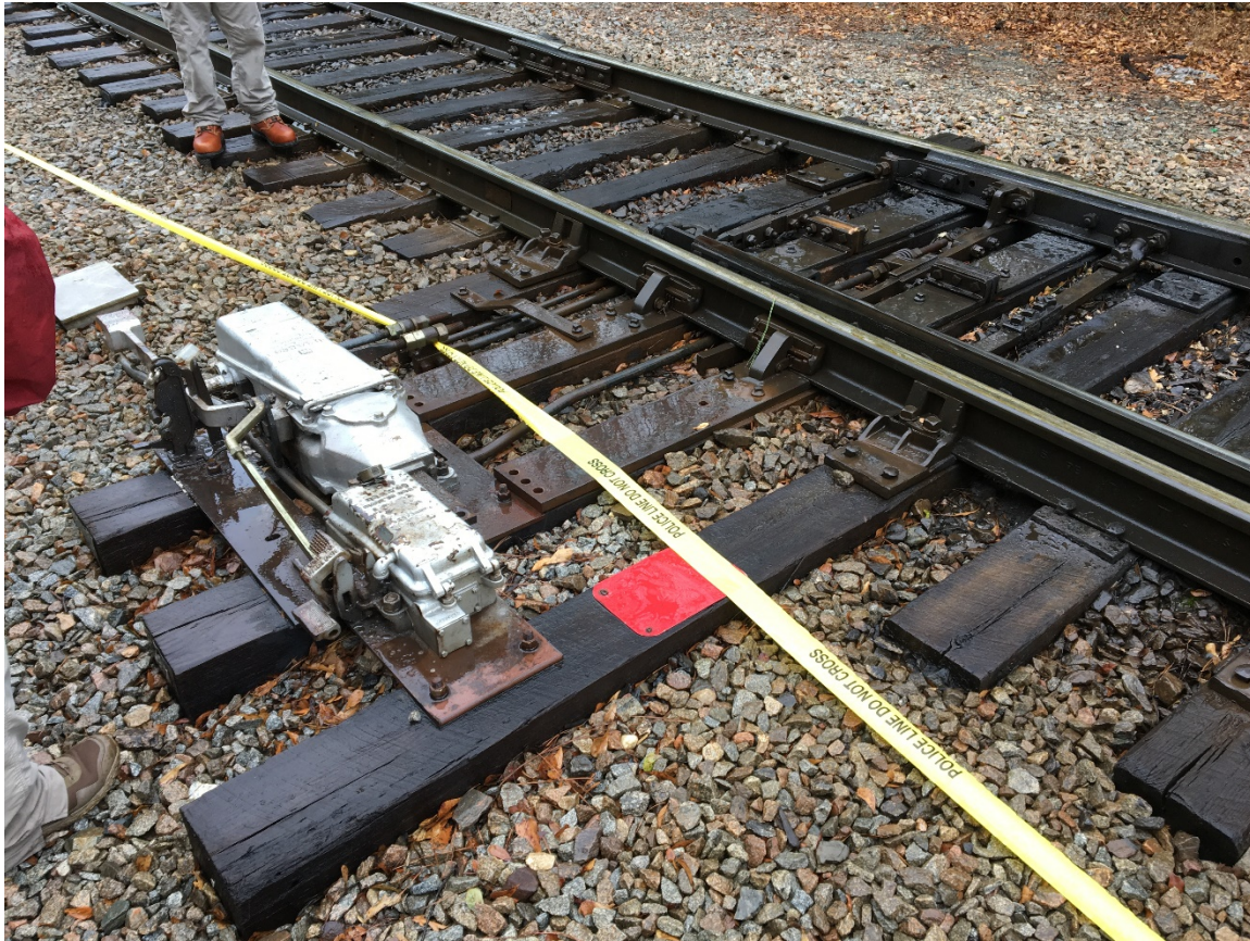
Figure 6. T21 hand throw switch with electric timeout.
