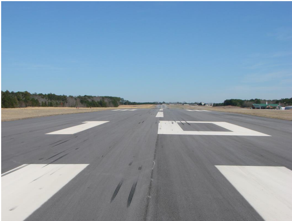
Photo 7: View looking down runway 10 during daylight (2/21/2013). 79
