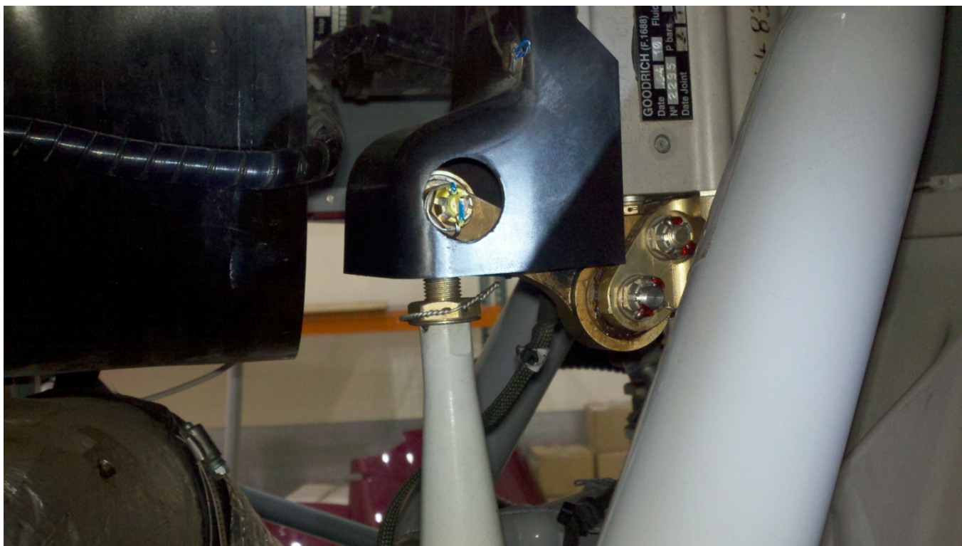
Fore-aft servo connecting hardware visible through the cutout of the ice boot (about eye-level for a pilot inspecting the left MGB area)
