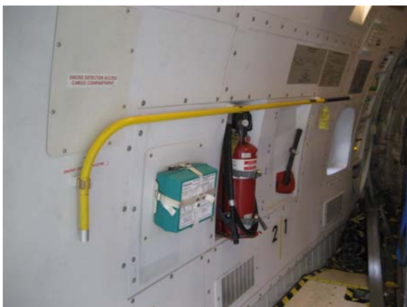
Figure 2: Main Deck Emergency Equipment
