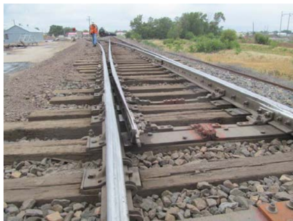
Figure 2 Switch points for track 141.
