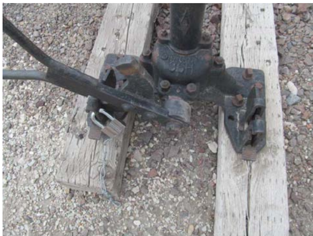
Figure 5 Switch stand and lock for track 740.
