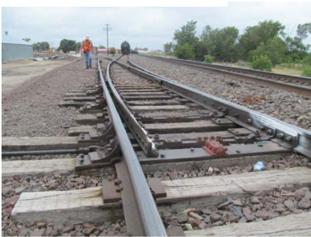
Figure 4 Switch points for track 740.
