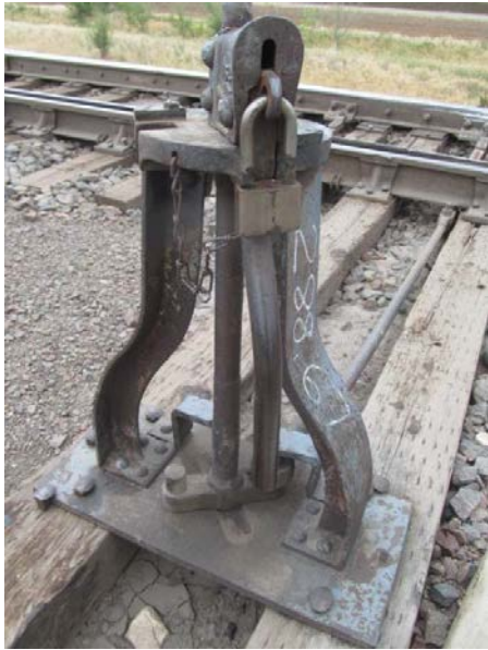
Figure 3 Switch stand and lock for track 141.
