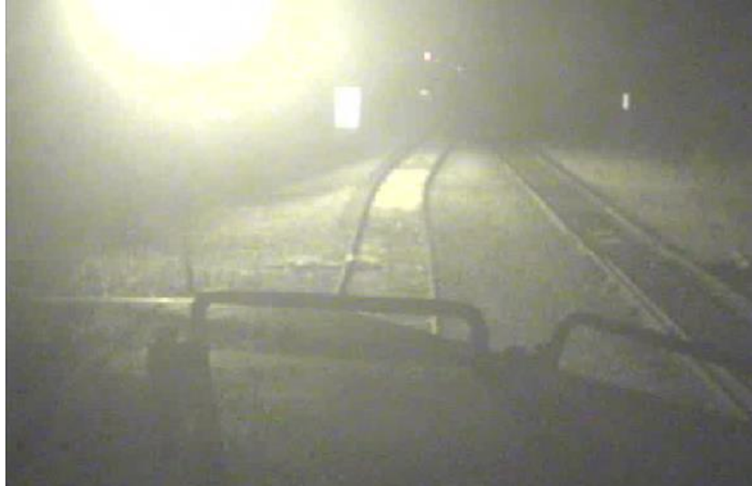
Figure 6. The derail and the position of the track switch.
