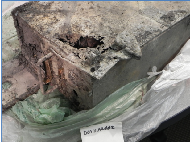
Figure 1. Fire damage to exterior of unit.
