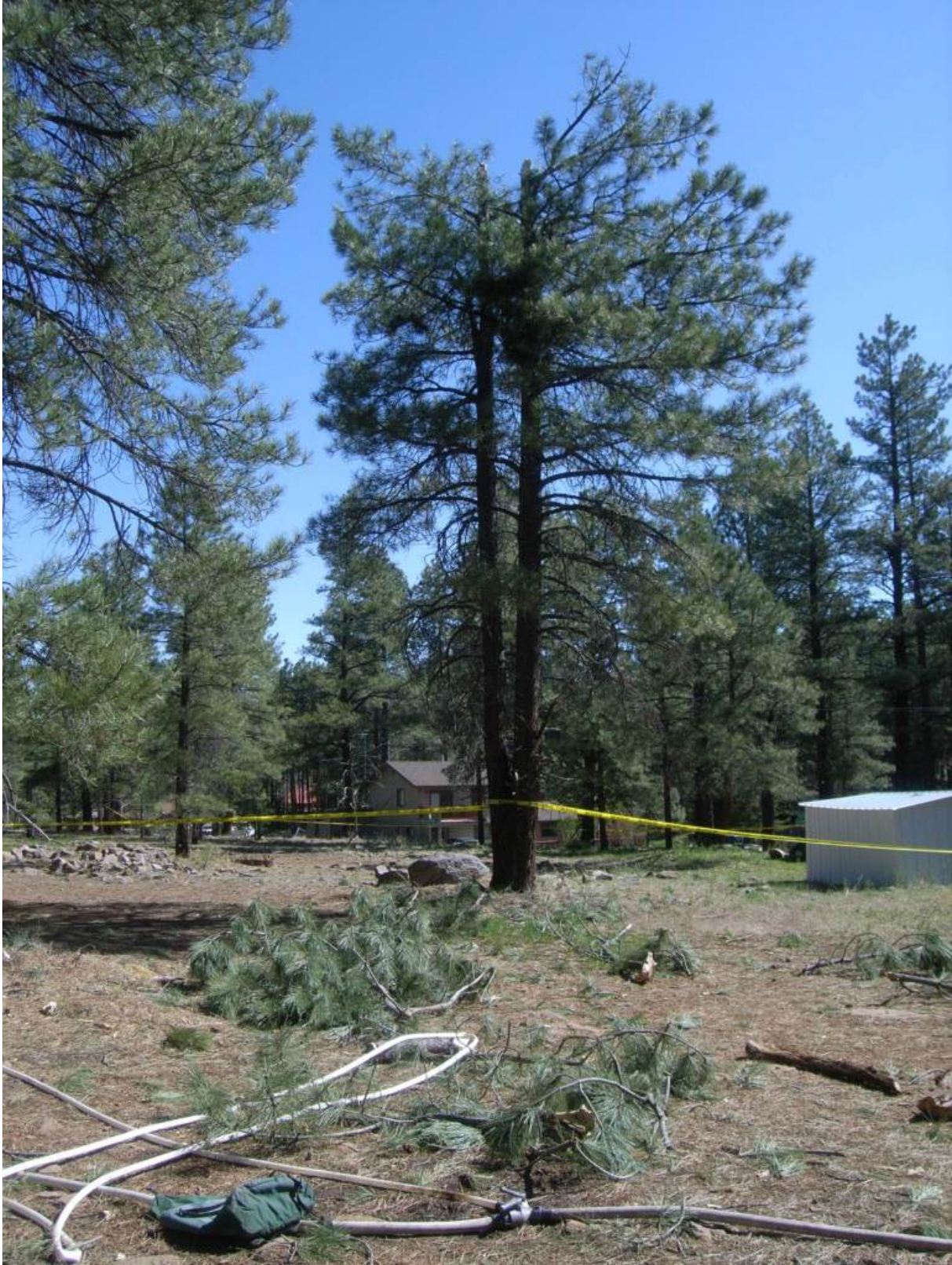
Figure 3 - Tree Strikes (View north)
