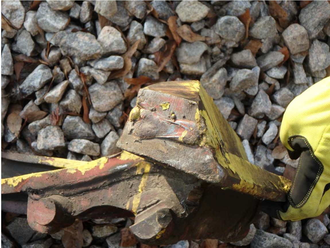
Figure 7. Photo showing the non-derailing end of the derail shoe with no indication of contact from railroad equipment.
