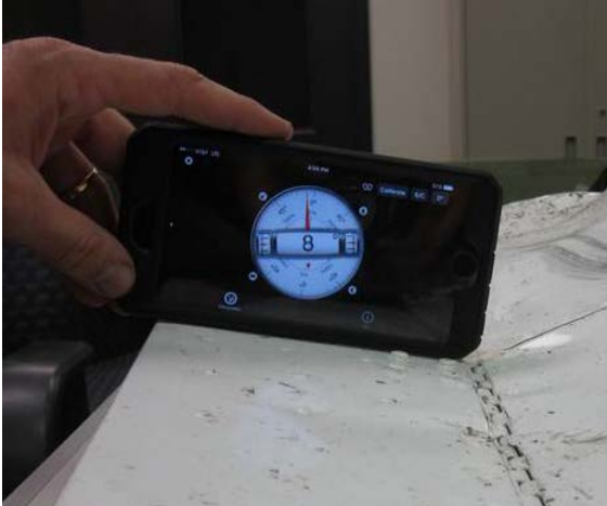
Photo 19 - Slope of tab. The tab deflection is about 30 degrees TEU. The pushrod was touching the bent portion of the elevator spar.
