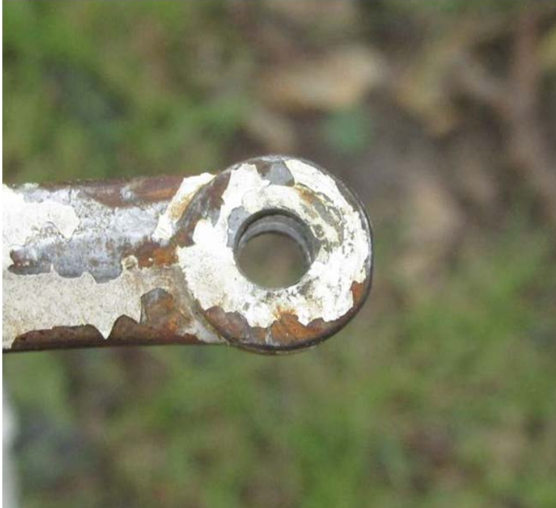
Photo 4 - Forward end of the pushrod. There was no apparent damage to the bolt hole (side one).
