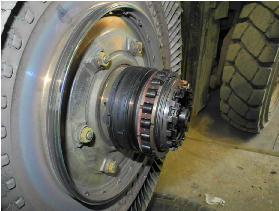
Rear LP Rotor Roller Bearing - Undamaged
