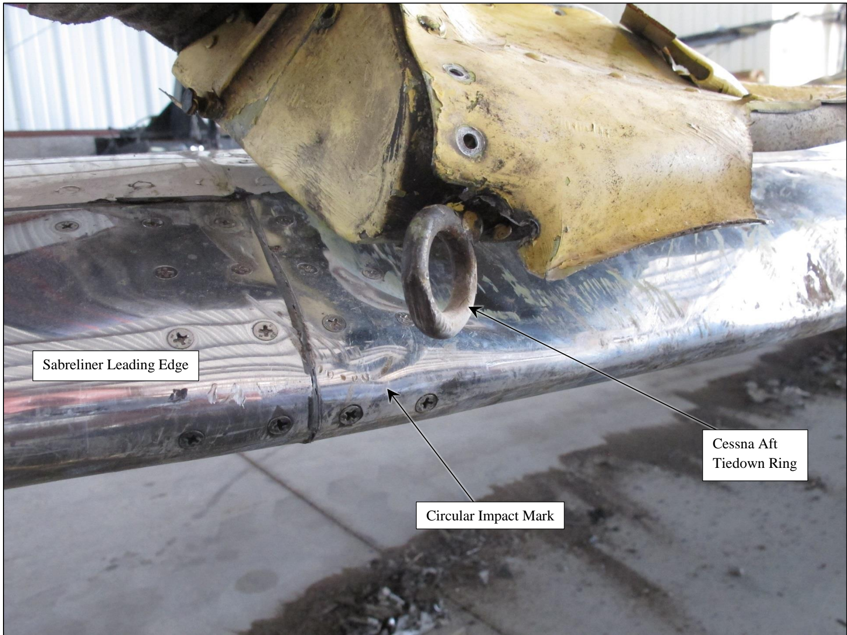
Photo 14 – Cessna Aft Tiedown Ring and Supporting Structure and Sabreliner Right Wing Leading Edge
