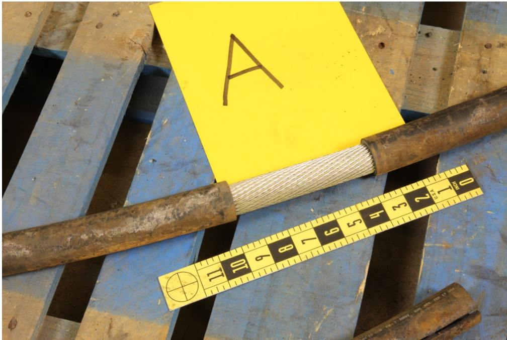
Figure 4: Portion of insulation removed from pig tail cable A.
