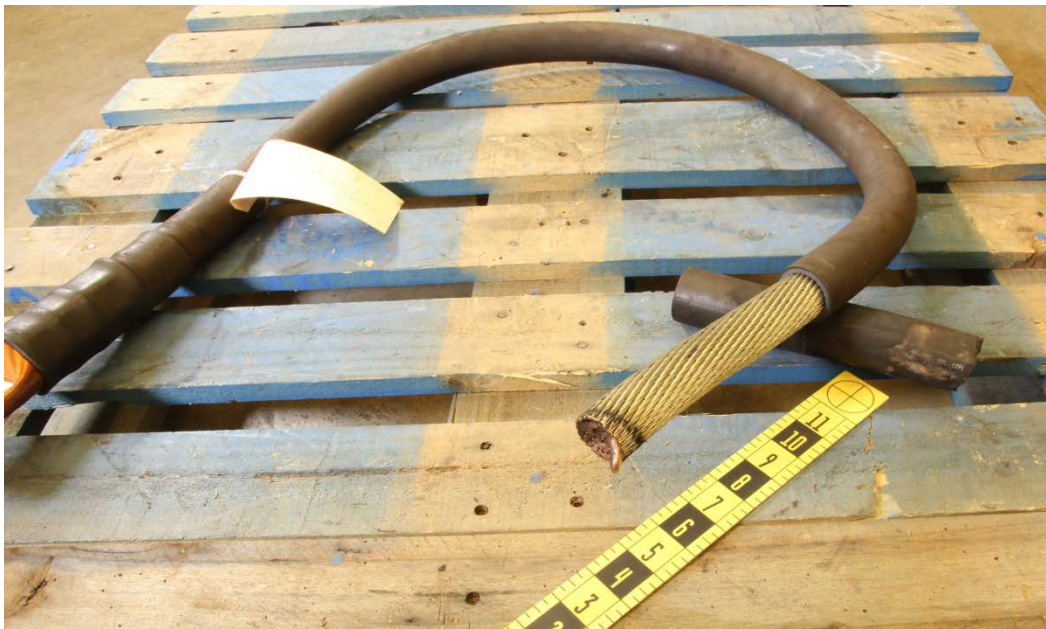
Figure 25: Fused end of South end pig tail cable with insulation removed.
