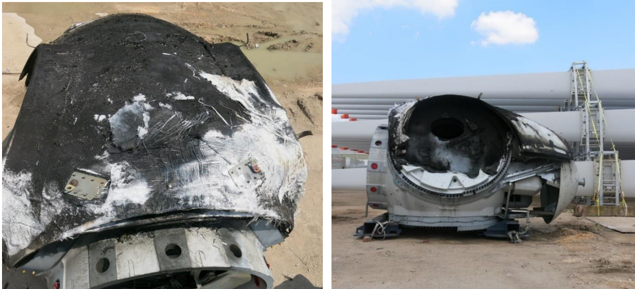
Fire damage to transmission hub as seen from above (left) and side (right) after removal from port cargo hold no. 3 of the Chipolbrok Moon .
