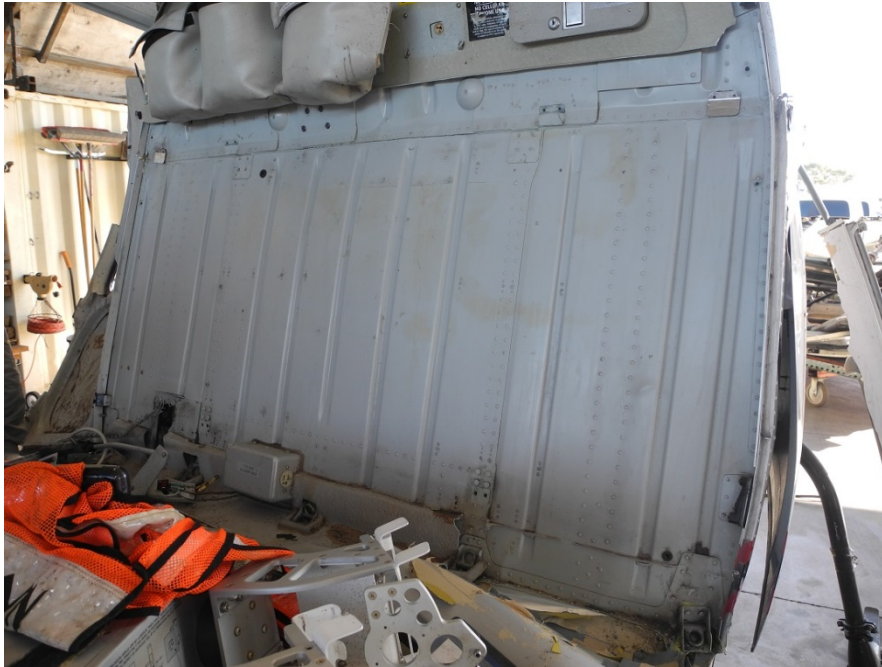
Photo 5. The aft vertical wall after removal of the lateral tracks, vertical straps, and wall cover.
