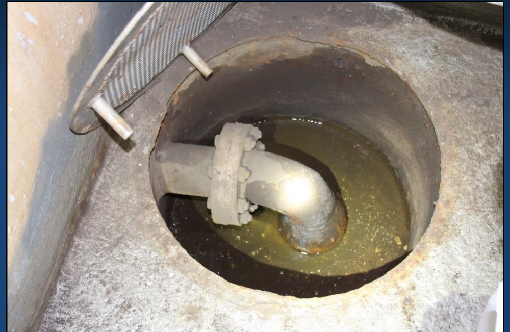
El Yunque Bilge Well, Hold 3
