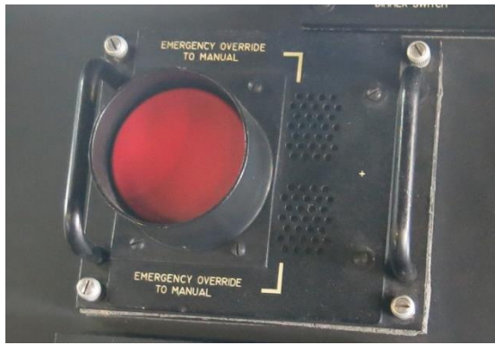
Figure 7. John S McCain emergency-override-to-manual button on the SCC.
