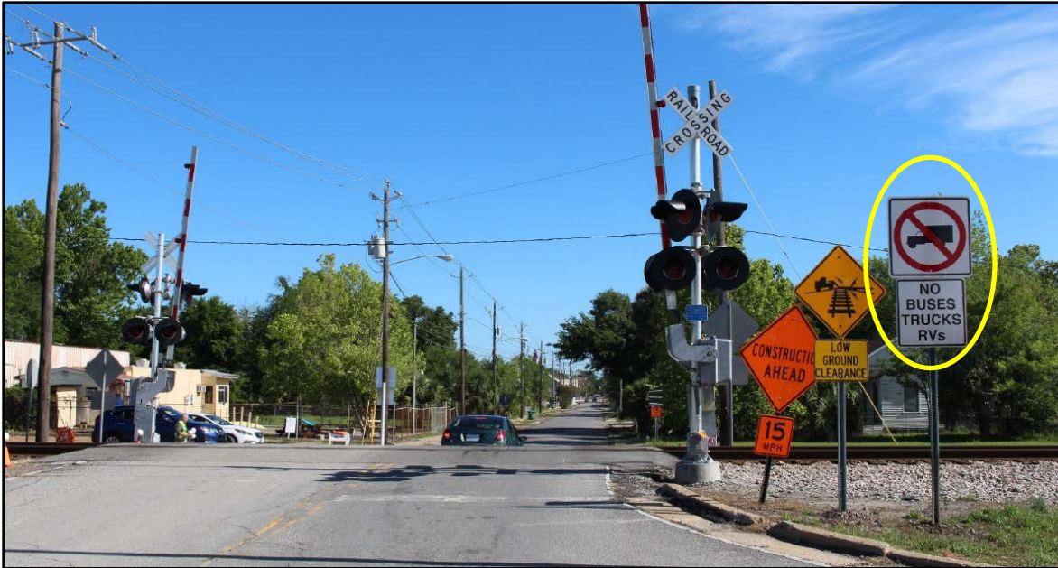
Figure 10. Postcrash view of the northbound approach to the Main Street crossing, showing the new vehicle exclusion sign and plaque (circled in yellow) posted by the City of Biloxi after the crash.
