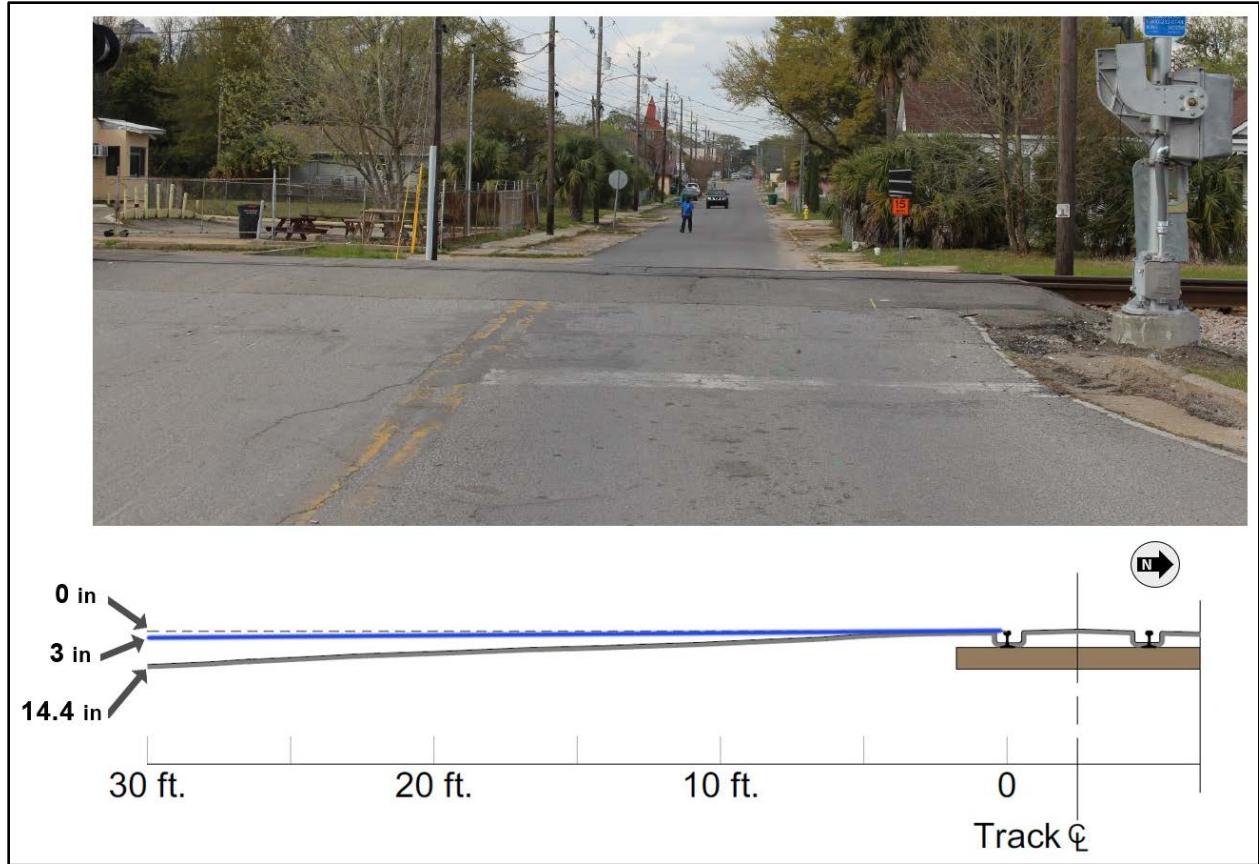
Figure 8. Photograph showing the northbound approach to the grade crossing (top)—what the driver would have seen—and cross-section diagram of the measured vertical profile of the approach’s slope (bottom). The blue line in the diagram represents the maximum elevation difference between the crossing and the approach as recommended by the FHWA and AASHTO, and the gray line represents the actual elevation difference at the grade crossing.
