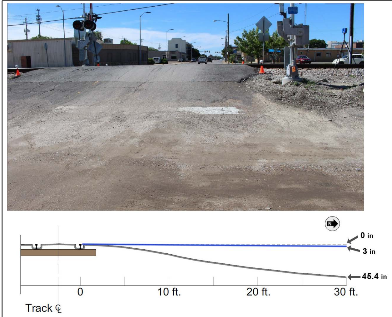
Figure 9. Photograph showing the southbound approach to the grade crossing (top) and cross-section diagram of the measured vertical profile of the approach's slope (bottom). The blue line in the diagram represents the maximum elevation difference between the crossing and the approach as recommended by the FHWA and AASHTO, and the gray line represents the actual elevation difference at the grade crossing.
