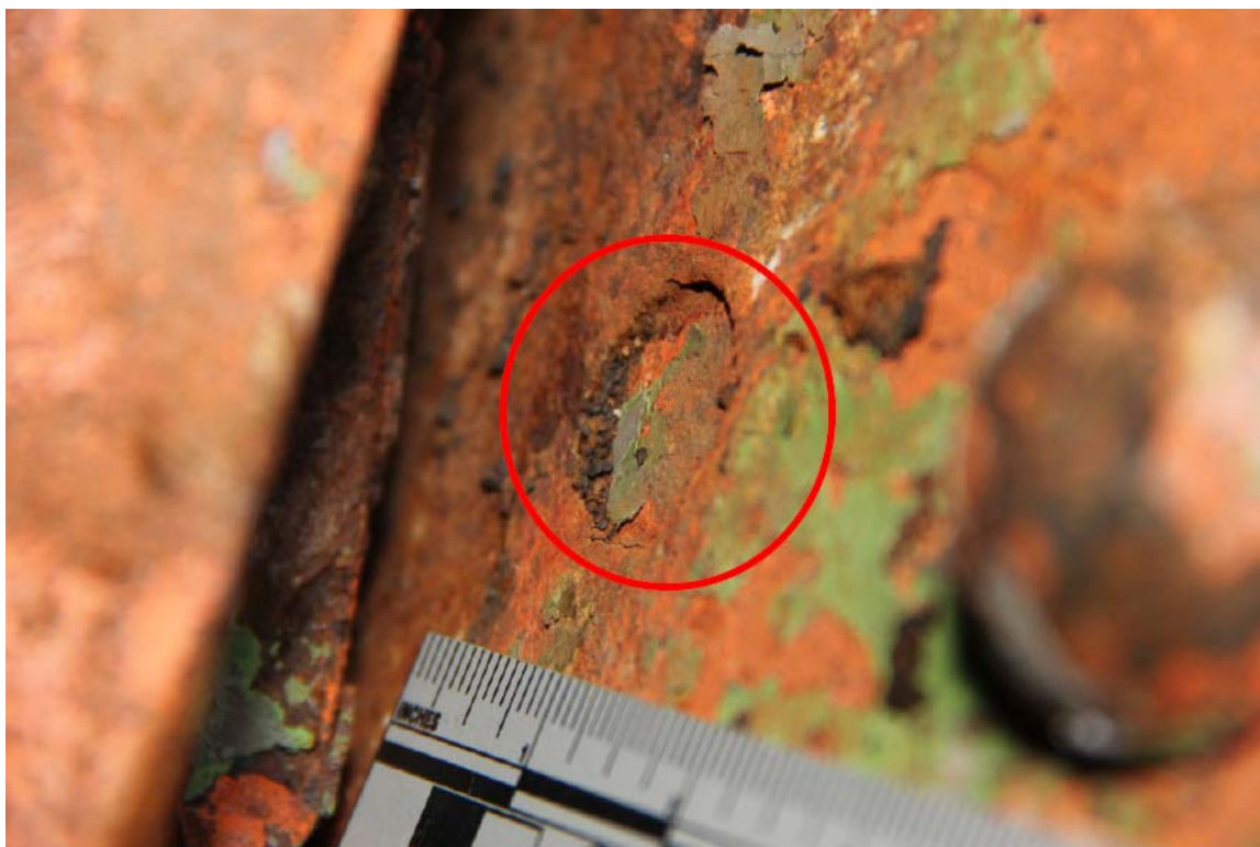
Photograph 7: Closer view of the rivet at the connection of U4W-L4W at the top of node L4W was cut with no connection to the mating material.
