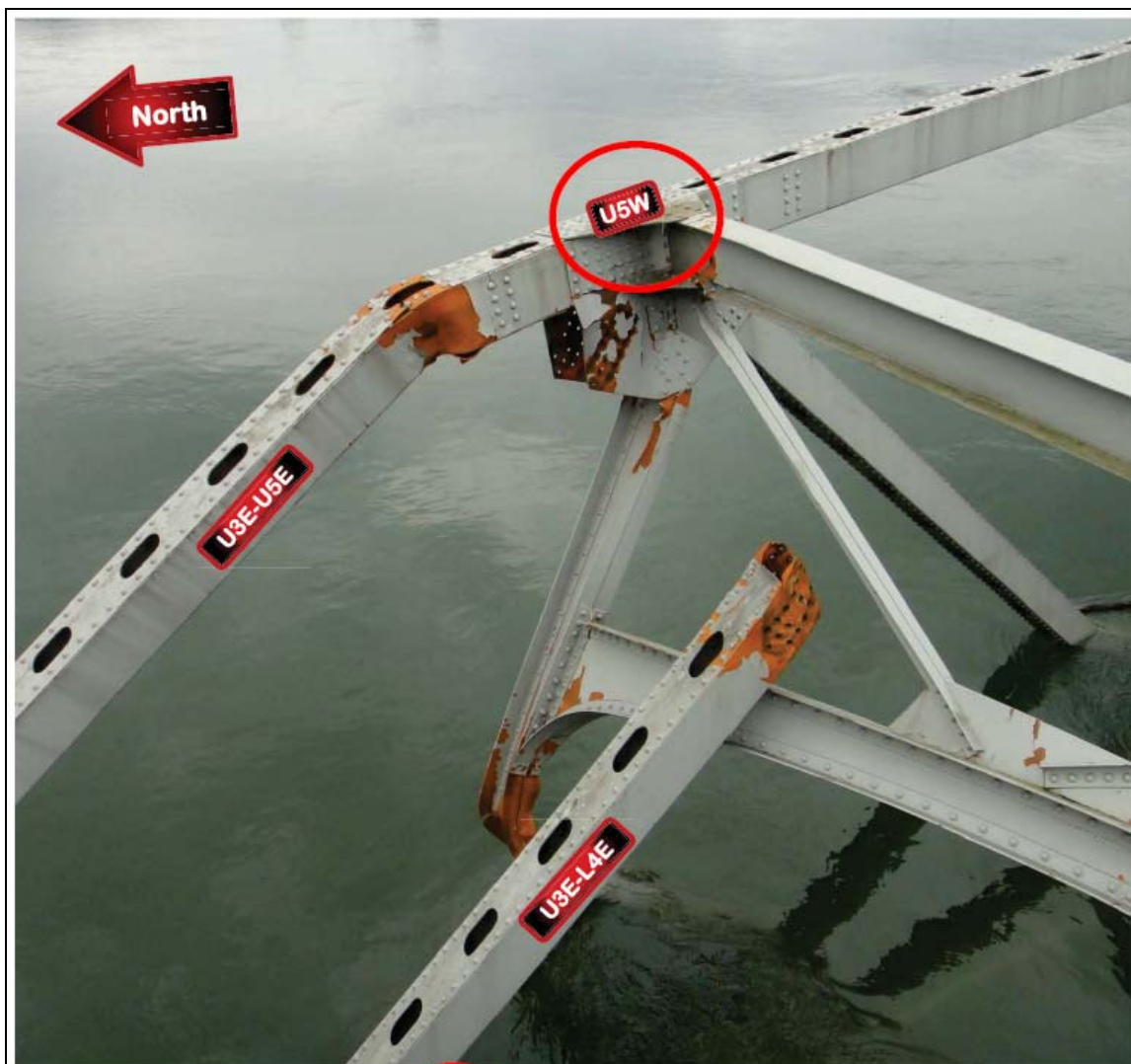
Figure 11. Node U5E with separated member U3E-L4E.
