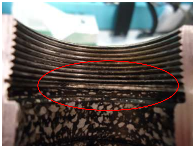
Figure 8. Damaged manifold threads (circled in red)
