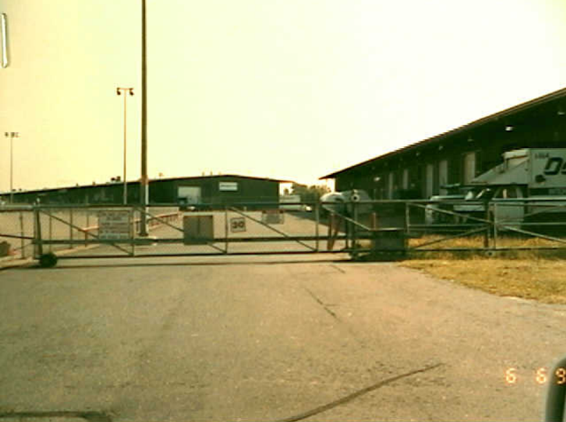
Meteorology 5 - Exhibit No. 5B - Attachment 56 - Photo 7. Airport view - Dobbs ramp and accident site.
