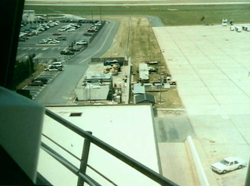
Meteorology 5 - Exhibit No. 5B - Attachment 56 - Photo 3. Camera 1 view.
