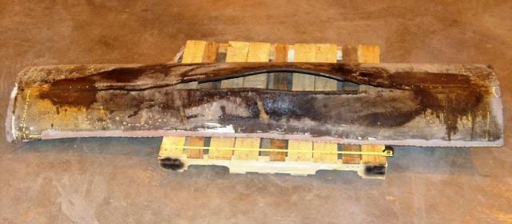
Metallurgical Group-Picture 20 Sample containing the rupture removed from the ruptured pipe piece at the NTSB Ashburn, Virginia Facility.
